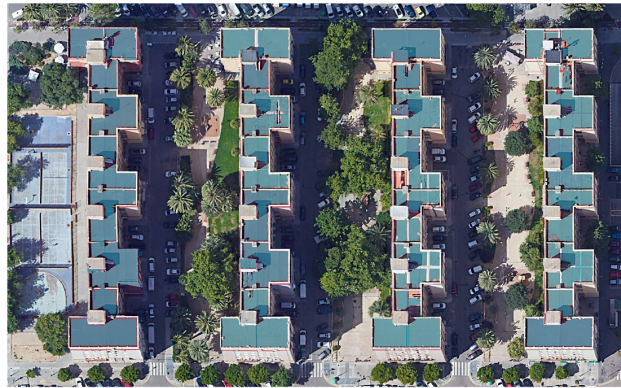
Figure 3.12: Final mask for roof detection. The original image is shown, and the resulting mask is overlapped onto it in a blueish colour. The base image is the cropped result of the GEP (LLC 2023) picture (2020) and the overlapped mask is produced using MATLAB (MathWorks 2022).
