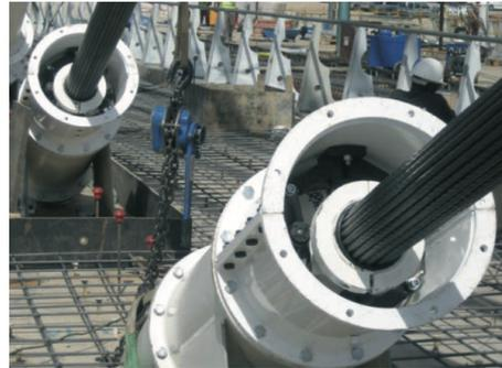
(a) Diagram of the anchorage of the cables
