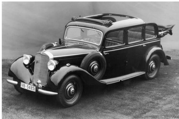
Figure 1.3. Mercedes 260D, first diesel production passenger car, 1936.
