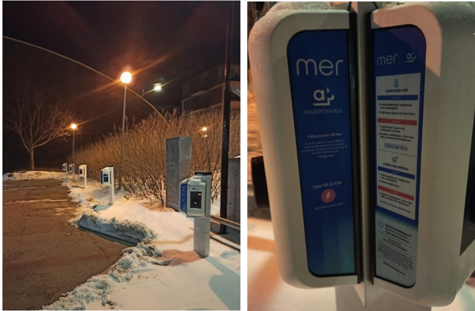
Figure 28. Pictures from Naturhistoriska CI, with 5 CSs, each delivering up to 22 kW.
