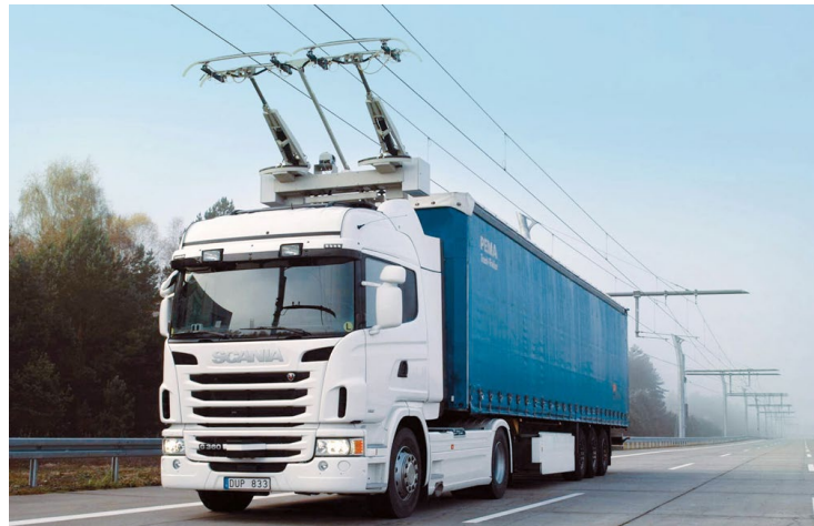
Figure 26. Siemens catenary system with pantograph connector on a Scania truck [101].
