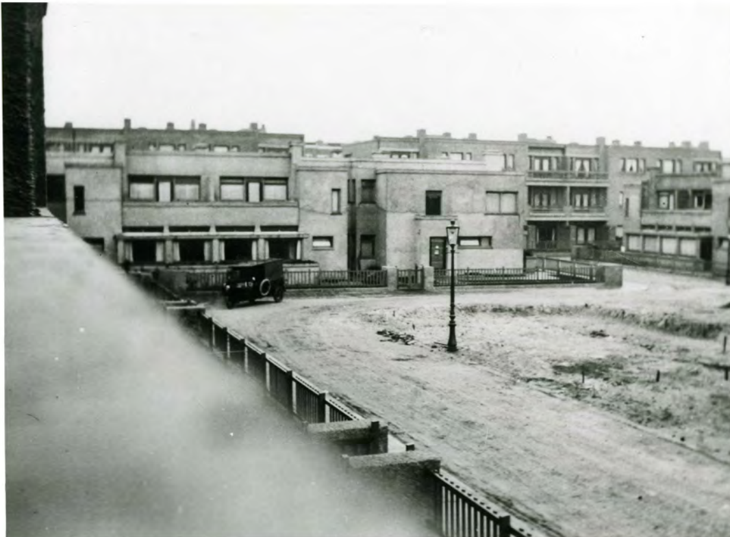
FIG. 21 Housing block by Jan Wils, Papaverhof, The Hague, circa 1921: Photo courtesy Marcel Theunissen.
