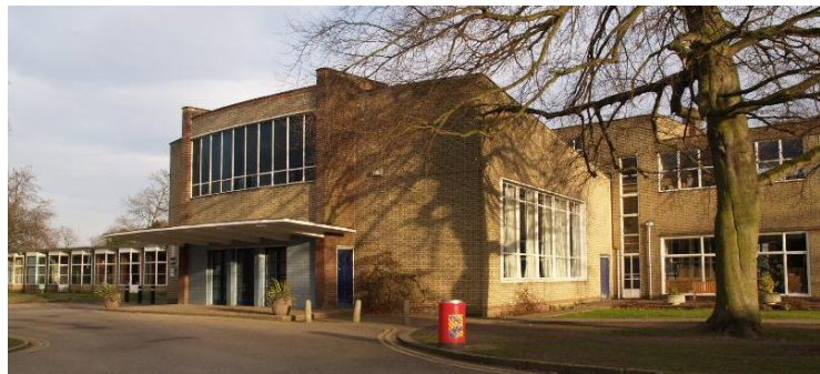
Figura 4. Foto exterior del auditorio del Impington Village College (Gómez Alfonso 2015, 188).
