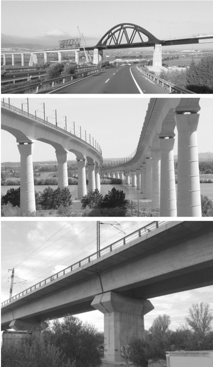
Fig. 10: Top: continuous concrete deck with arch over the motorway Granada–Seville (Spain). Image courtesy of José Lavado Rodríguez ( http://hlestructuras.com ). Middle: double viaduct over the Rhône river in Avignon (France). Image courtesy of Philip Bourret by way of structurae.net . Bottom: simply supported spans on the Madrid-Barcelona high-speed line (Spain) with pre-fabricated concrete beams.
