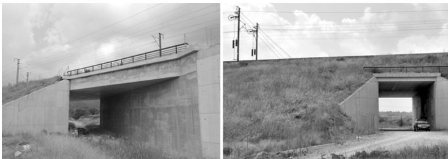
Fig. 12: Skewed (left) and straight (right) rigid portal frames. Madrid-Valencia line (Spain).
