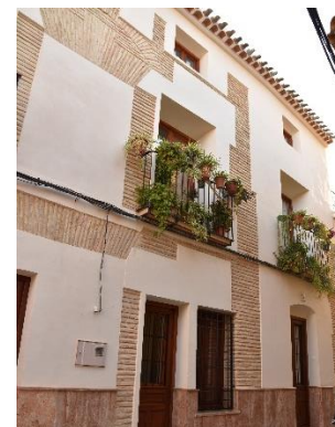
Very good No presence of cracks nor moisture
