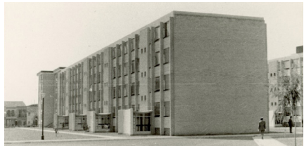
Figure 5. View of the block in a photograph from the 1960s. Source: (IVVSA Archive)
