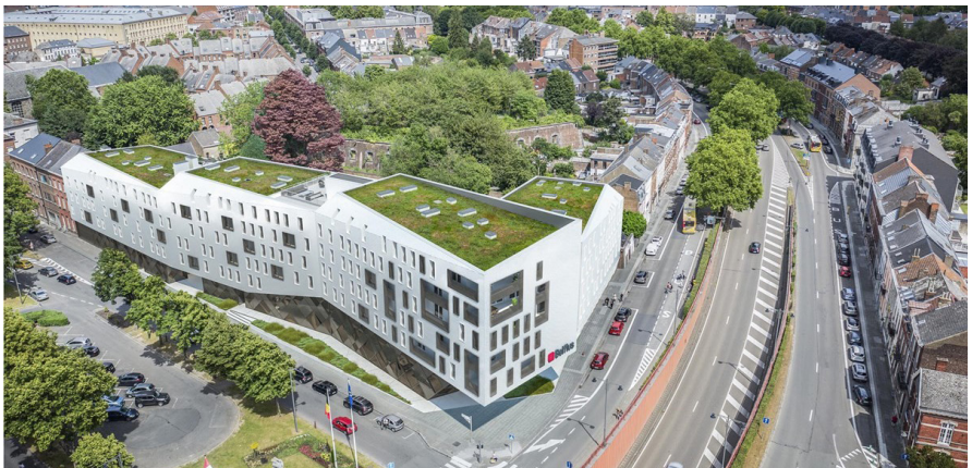
Figure 1: Proposal for the mixed building (housing, offices and kindergarten) of the regional headquarters of the bank Belfius, Avenue Jean d'Avesnes. Mons, image arch. NOHO, Brussels, 2019
