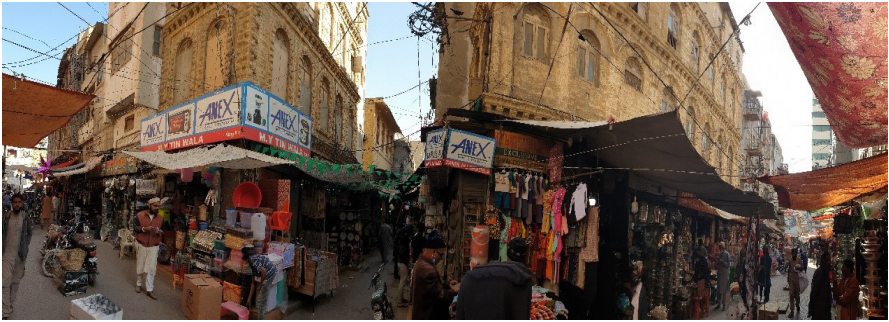
Figure 4. Panoramic Street view of Bohra Street in Bohri Bazaar showing the condition of British era buildings and multi-functional activities going-on in the area. Source: Images taken by Syed Hamid Akbar( First author) during 2020-2021 fieldwork
