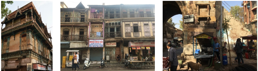
Figure 1. Abandonments and encroachments in the Walled City of Ahmedabad This situation in the Indian historic districts highlights how the definition of specific guidelines for preserving the traditional buildings of the historical fabric, which can be incorporated into the future change of cities, is still weak. (©Authors 2019)
