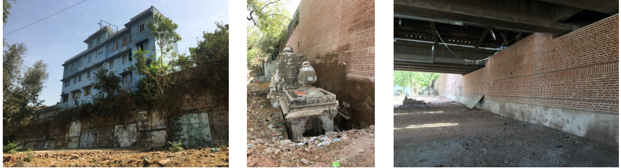
Figure 5. Encroachment along the city wall: new constructions along the historical walls (left), scarce consideration of historical pre-existences such as temples (middle), demolition of the walls for new infrastructures (right). It is noticeable how – paradoxically - the sense of authenticity is preserved where the walls have not (yet) been the “victims” of renovation work (left), while the historical patina has been totally lost with the incongruent rebuilding of the wall (middle and right). © authors 2019
