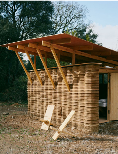
Serra Utkum Ikiz. 12/09/2022, Spain's first building made with earth and a 3D printer: TOVA
