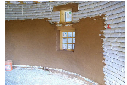
@brandonv111, 2018, Earthbag Construction Building a Cheap and Environmentally Friendly HomeSteemit
