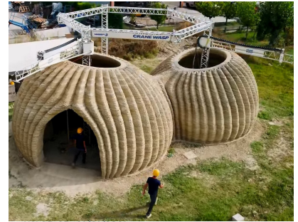
WASP 3D, 21/01/2021, Eco-sustainable 3D printed house min: 1:33
