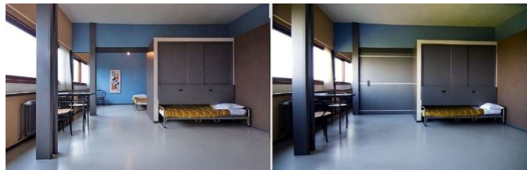
Fig. 2. Elements of day/night-time adaptability in the Stuttgart houses: sliding partitions and closet with wardrobe and sliding bed.
