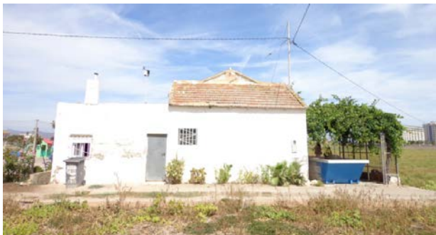
Figure 1. South building façade.
