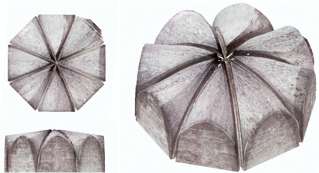
Figure 3 | Point cloud containing 7,085,550 points of the vault of the Sacristy Mayor of the Metropolitan Cathedral of Valencia.
