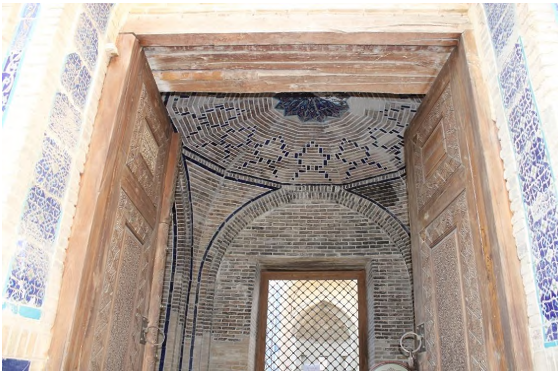
Source: Author: gate and roof of entrance
