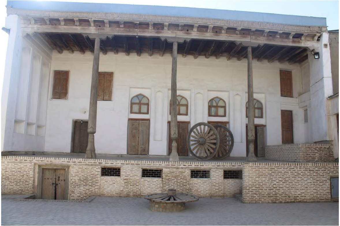
Source: Author – outer courtyard and ayvan
