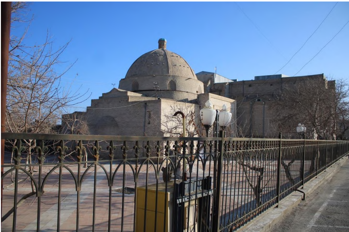
Source: Author: backside of the Mosque, it is surrounded by iron barrier
