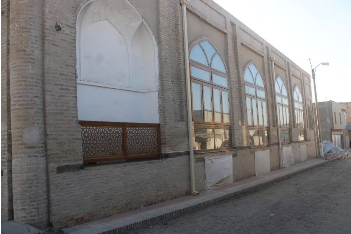
Source: Author: The northern walls and street road.
