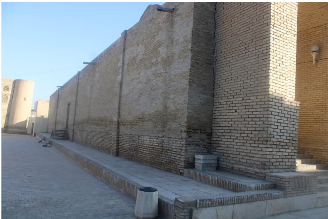
Source: Author: The south walls of the the Trading dome. Possible to see the affect of the humidity
