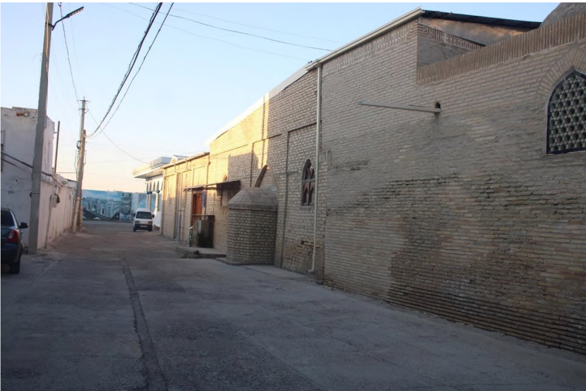
Source: Author: Western walls and street
