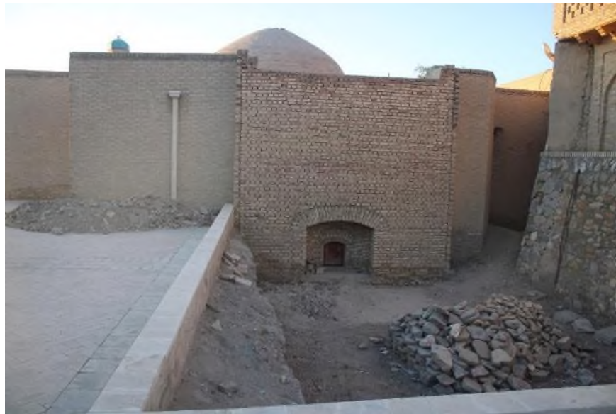
Figure 38. South part of the hammam Sarrafon
