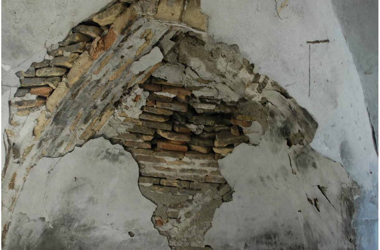
Source: Author: Inside the building, roof part.
