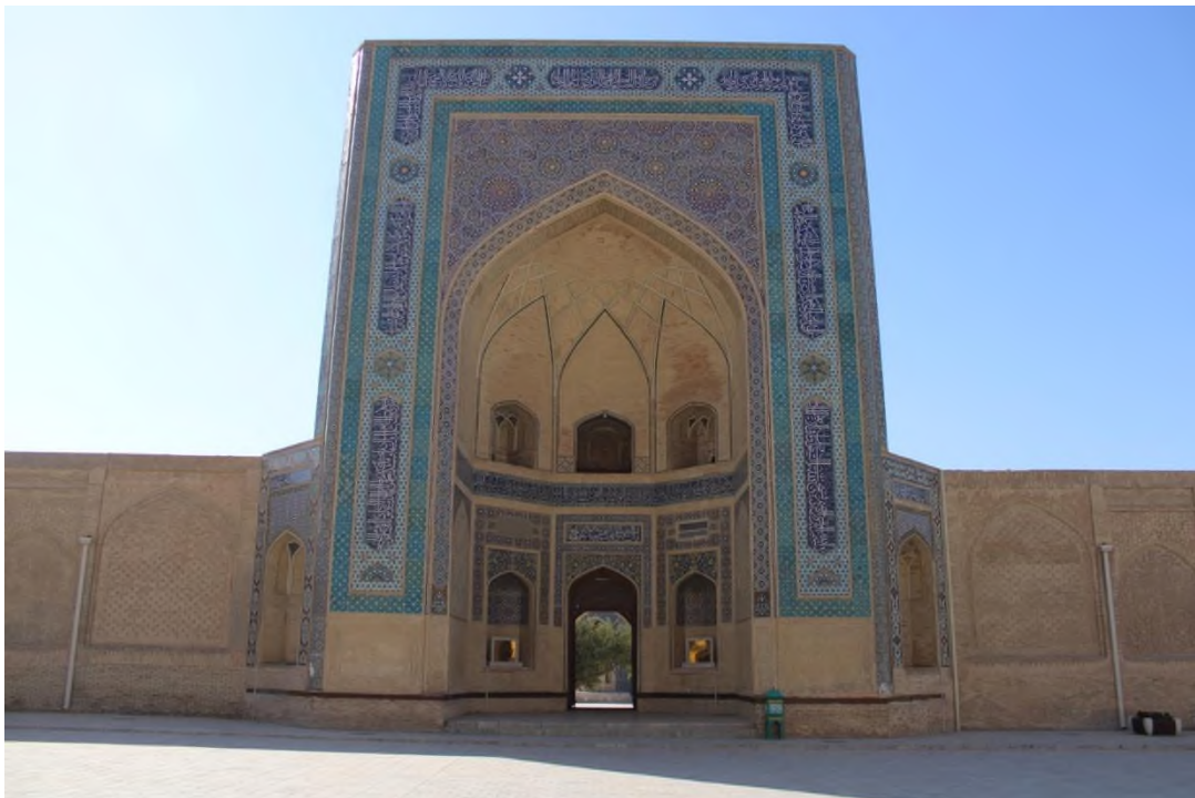
Source: Author: The Eastern gate of Kalyan Mosque.
