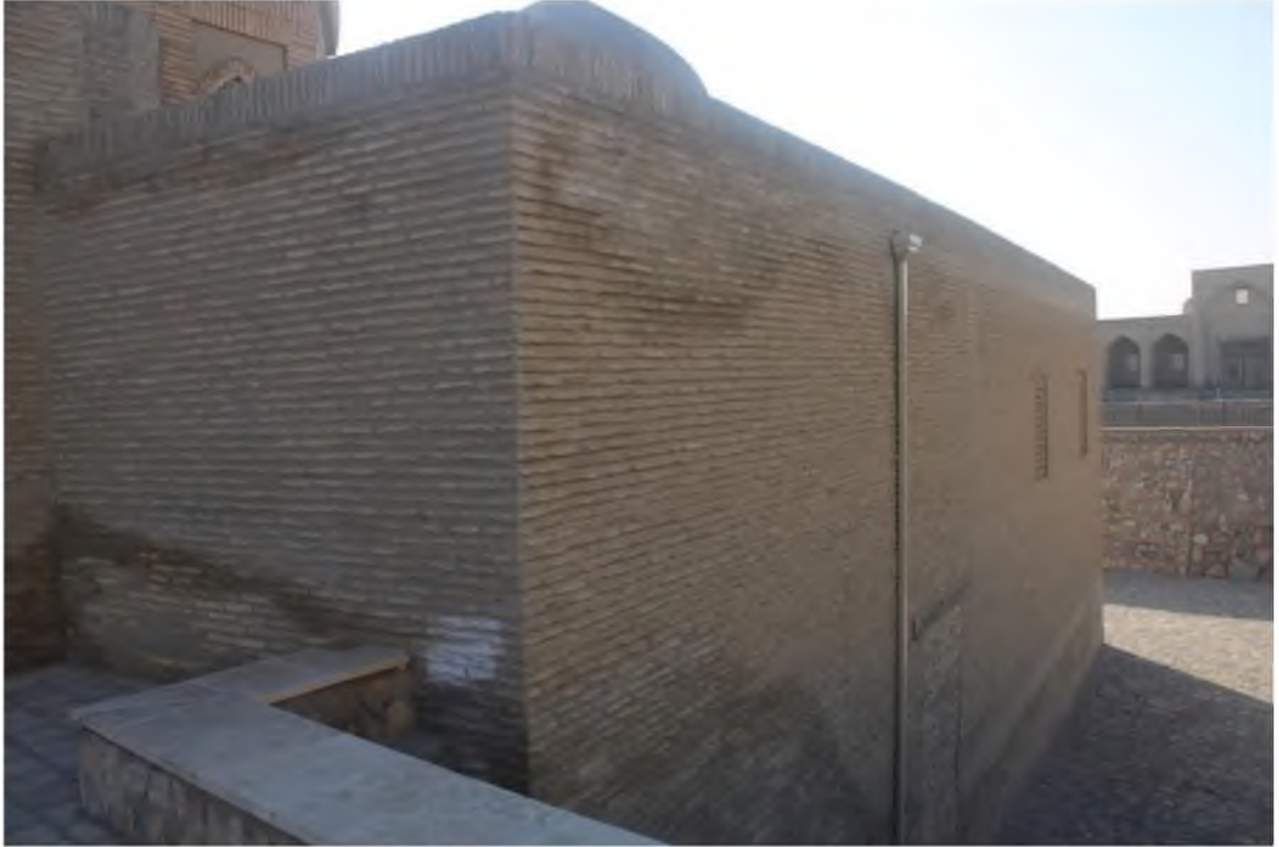
Source: Author: picture from northern-east part. Could see the effect of salinity and deem.
