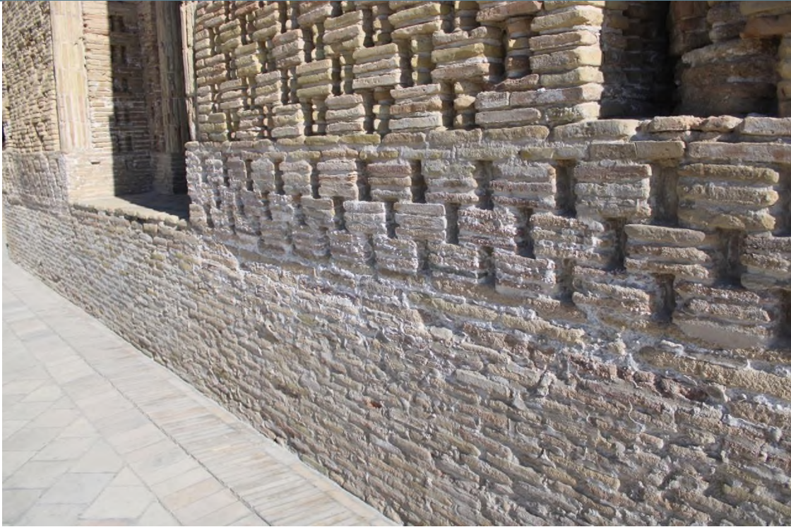
Sources: Author: Affect of salinity and humidity on the fundament of the walls
