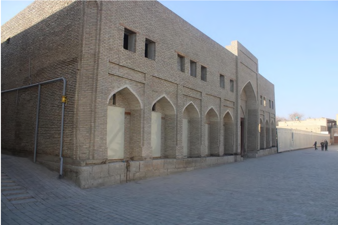
Source: Author: view from the front side after reconstruction works of Rashid Caravansarei
