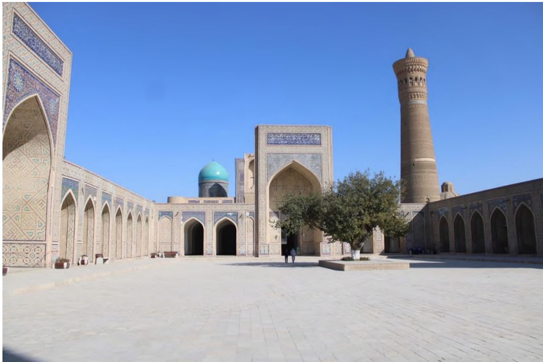
Source: Author: Inside the Kalyan Mosque
