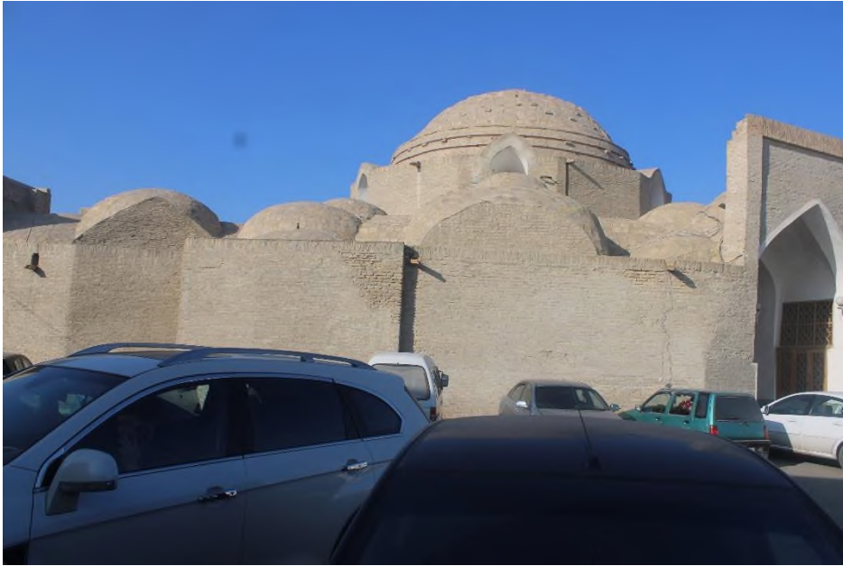
Source: Author: view from the south of the building
