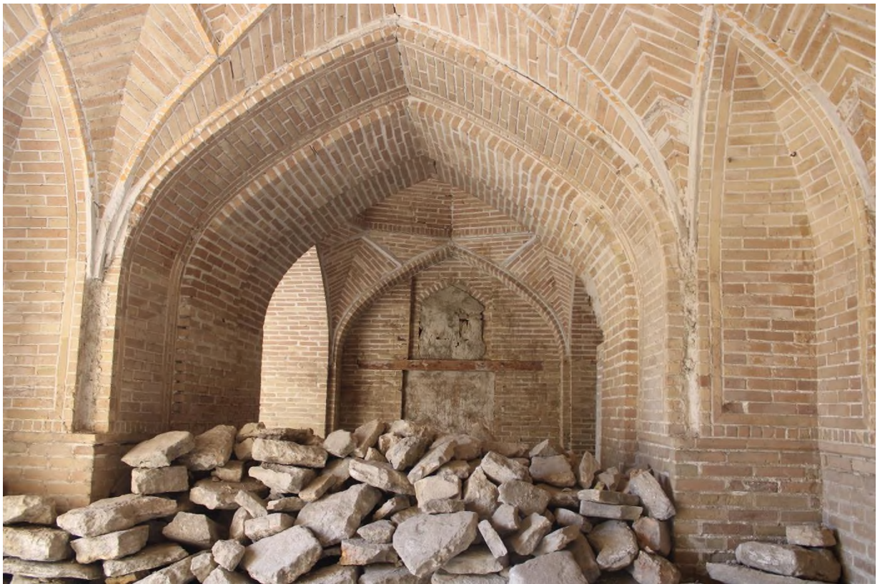
Source: Author: inside the built heritage.
