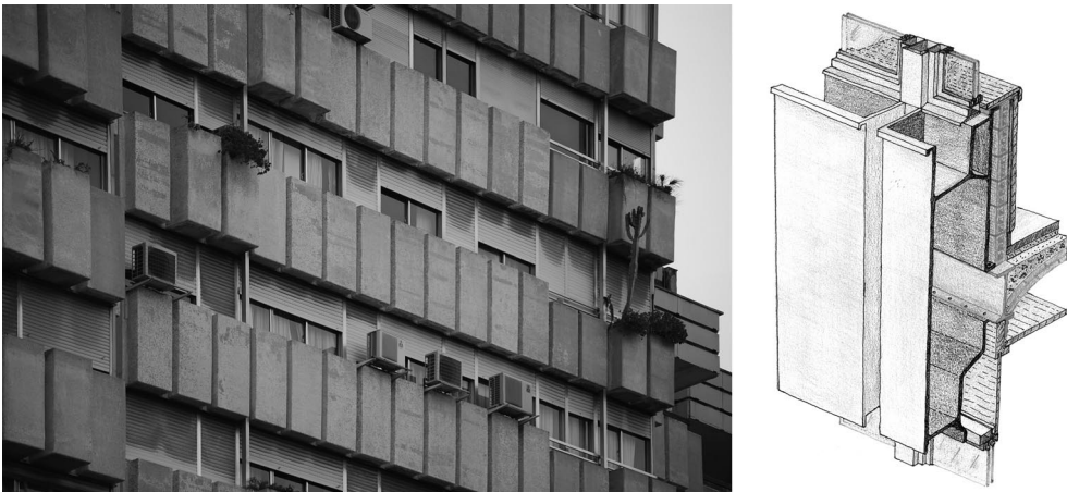
Figure 6 left. Detail from prefabricated facade elements. Asbestos-cement Modular boxes. The vegetation integrated into the facade can be clearly seen. Luz building. Valencia. Architect, GO.DB. Architects. (Photo: Maite Palomares, 2009. Private Archives of Maite Palomares.)
