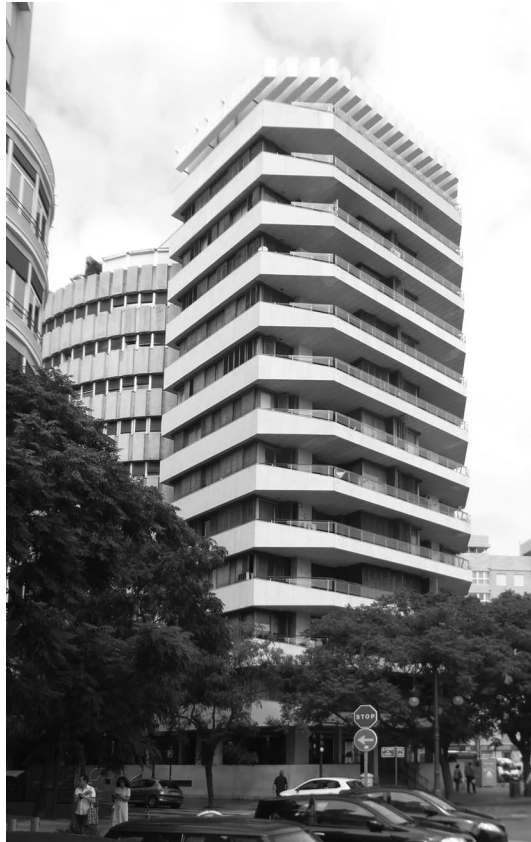
Figure 9. General view of the front of Sorní Building. Roof topped with a pergola of a section similar to the Modular Boxes of the Curved façade. The balcony ledges of variable section characterize the main façade. The horizontal composition predominates as a whole despite the verticality of the Modular Boxes. Valencia. Architect, GO.DB. Architects. (Photo: Maite Palomares, 2009. Private Archives of Maite Palomares.)
