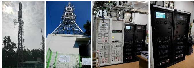
Fig. 2. Transmitter facilities of the Seoul Metropolitan SFN.
