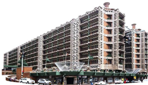
Figura 3. Complejo comercial y de oficinas Eastate Center, Harare, Zimbabue. [imagen digital]. Fuente: https://www.livinspaces.net/ls-tv/watch-how-the-eastgate-center-in-zimbabwe-cools-itself-without-air-conditioning/
