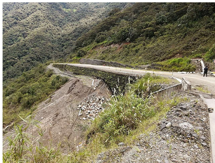
Figure 2. A view of the middle part of the landslide area where the road was affected (cut) and reconstructed, applying observed earth-walls. In this location, the movement is prone to continue at a low displacement rate. The high slope on the landscape can be observed.
