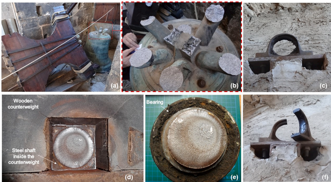
Fig. 2. Photos taken after the collapse of the bell.
