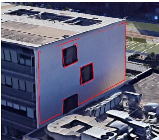
Figure 20. Building 4P West facade surface consideration.
