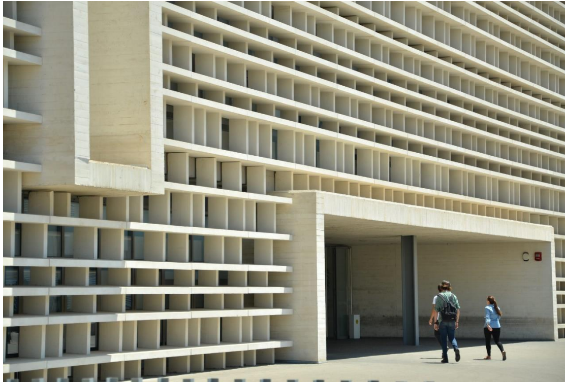
Figure 19. South facade of the building 4P.
