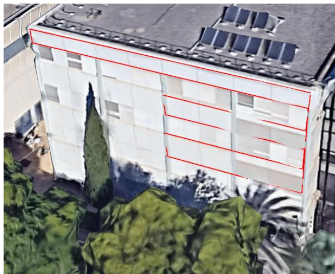
Figure 18. Building 5E, left side, South facade surface consideration.
