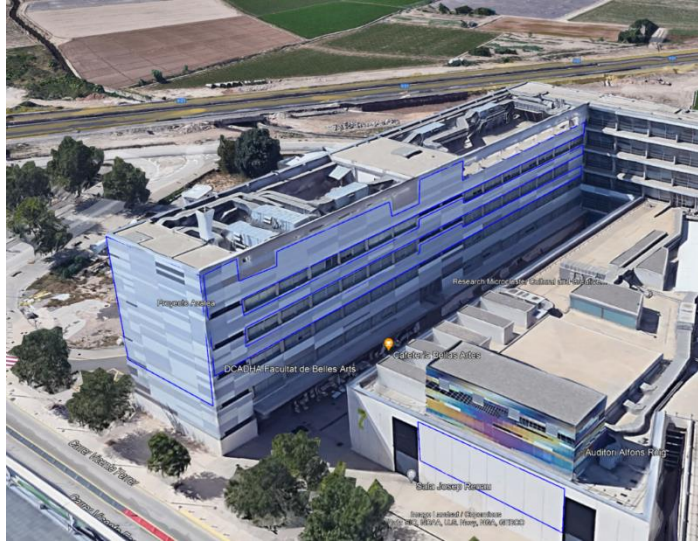
Figure 16. Façades Surface measurement for building 3N
