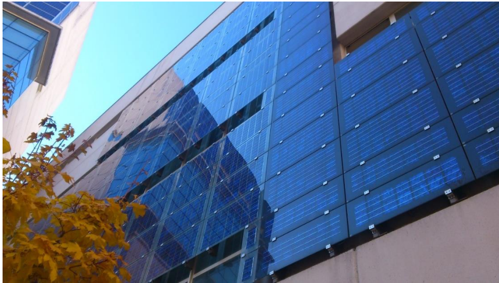
Figure 9. BAPV façade configuration. [19]
