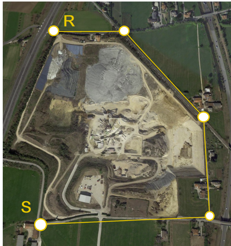
Figure 12. Positioning of nodes in quarry test.
