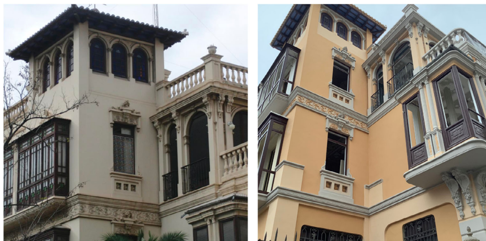
FIGURE 1 Left: Exterior of Palacete de Burgos (1921), an eclectic building by architect Javier Goerlich Lleó, Valencia (Spain). Photo August 2020. Right: Exterior after restoration of the original colors by GICA-UPV, with the grayish color of ornamental elements emphasized on the ocher background; architectural project by Javier Hidalgo. Photo: 2021.
