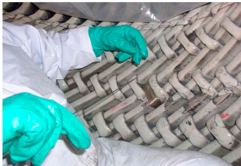
Figure 2. Restating ties with glass roving and resin.
