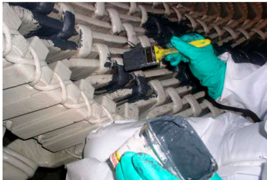
Figure 4. Painting of the restored area with resin.
