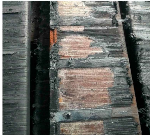
Figure 1. Electrical Erosion (2012)—Stator Bars.
