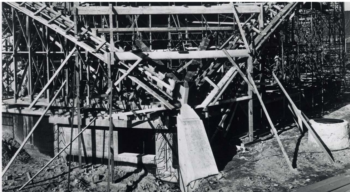
04. 22 E. Eero Saarinen. Kresge Auditorium, MIT Boston (1954-55). Encofrados cubierta (1953) © Eero Saarinen Collection (MS 593). Manuscripts and Archives, Yale University Library. Series IV. 32274668
