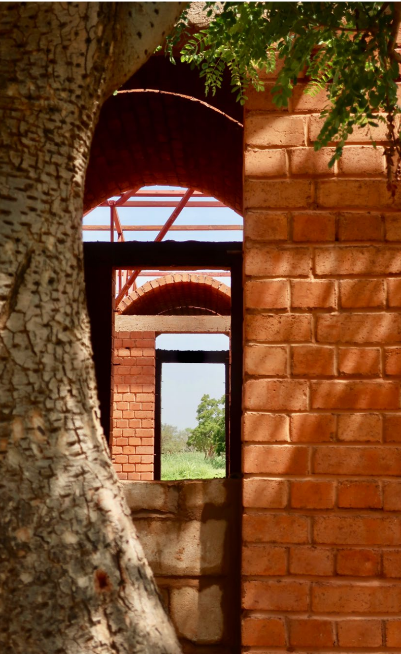
Administration building under construction, Phase 2 of the project.
