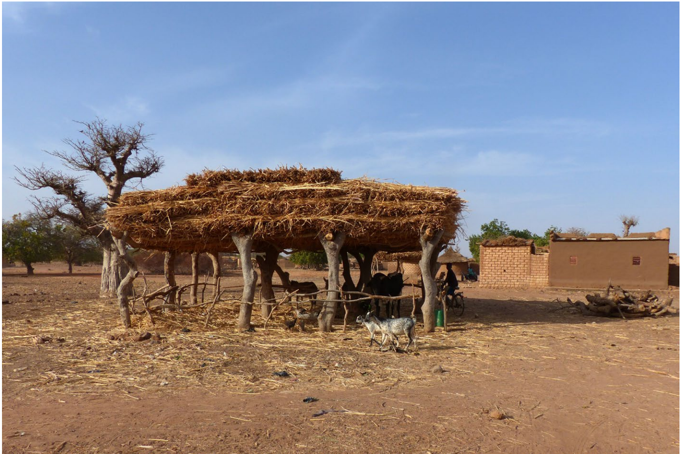
Shed with straw stored in intercrossed layers on the roof and used simultaneously as a goat pen.
