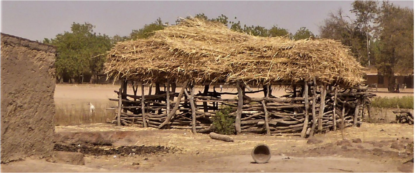
Shed surrounded by a small log fence.
