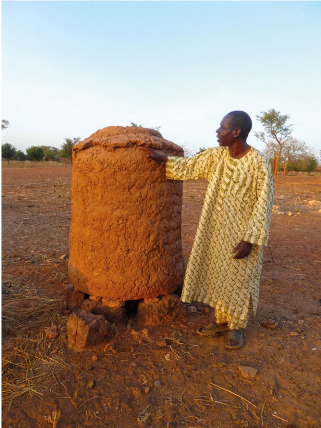
Old Mossi silo built with termite nest earth.
