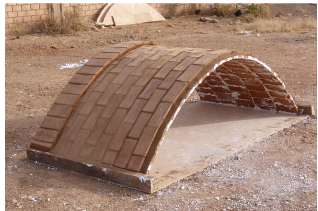
A finished vault in the Ouagadougou workshop.
