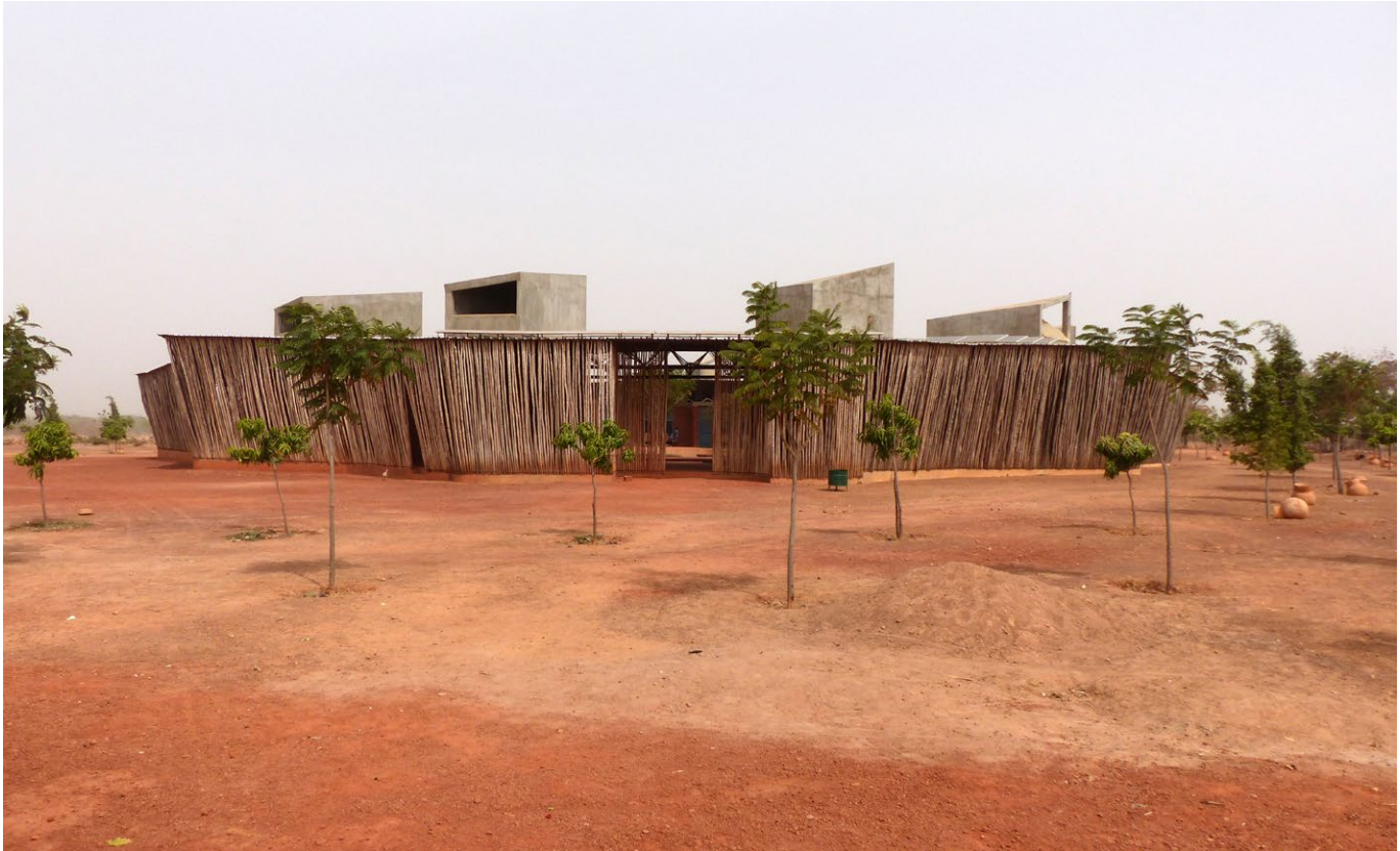
Schorge Lycée in Koudougou, designed by Francis Kéré.
