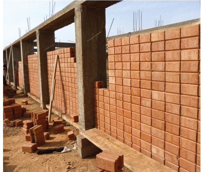
Construction of a CEB enclosure in Ouagadougou, Burkina Faso.
