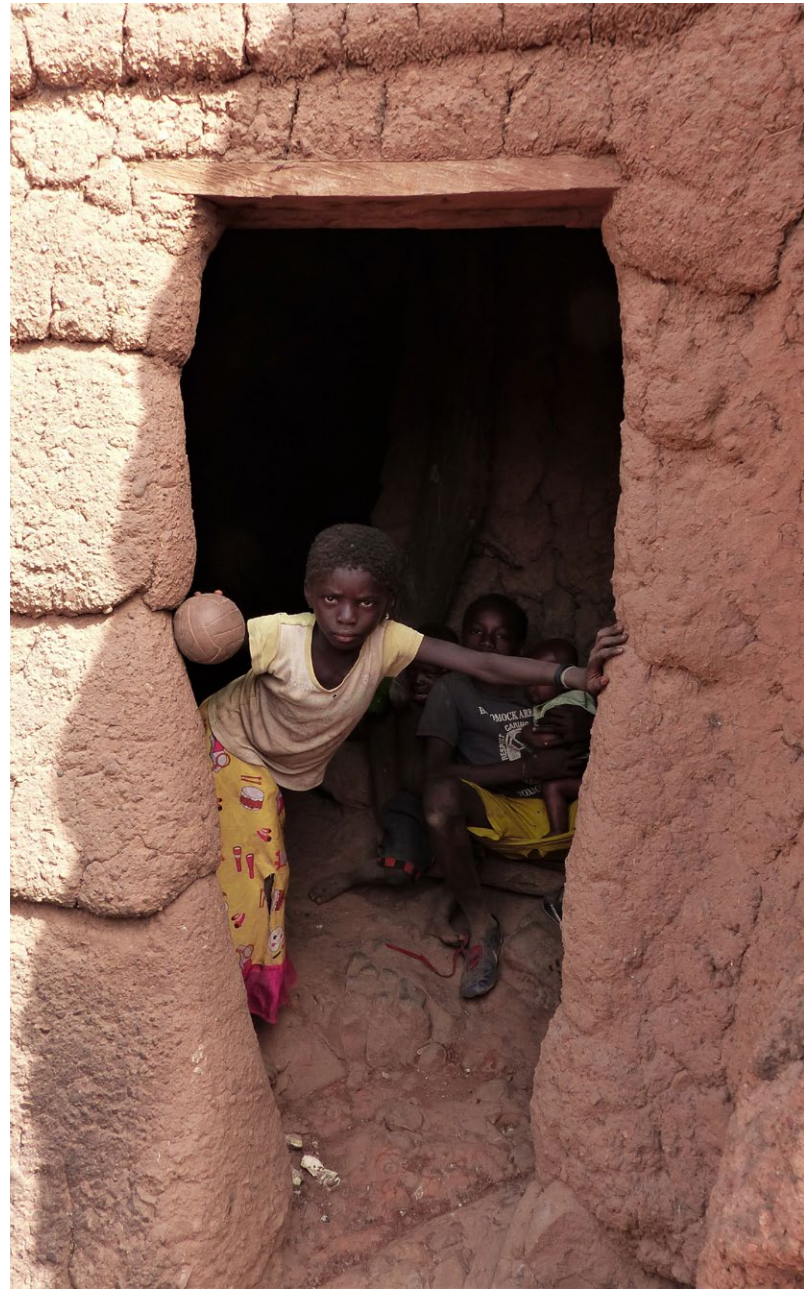
Tapered opening with a lintelled access to the Lobi dwelling.
