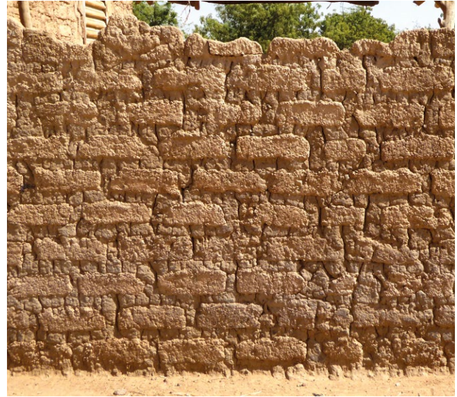
Adobe construction bonded with clay mortar.
