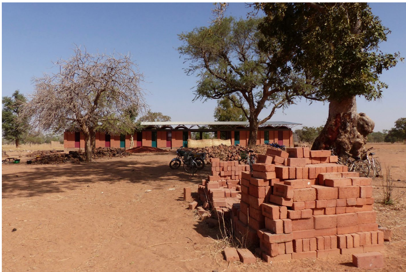
CEBs stored outside the school ready for the next construction phases.
