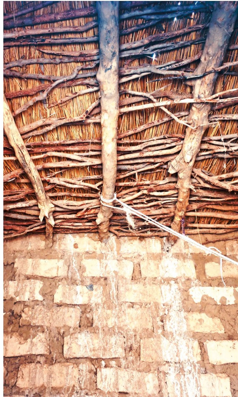
Inner view of a traditional roof.
