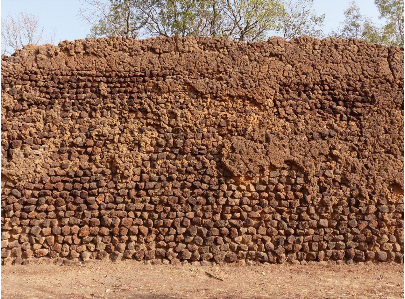
Laterite masonry wall in Loropeni.
