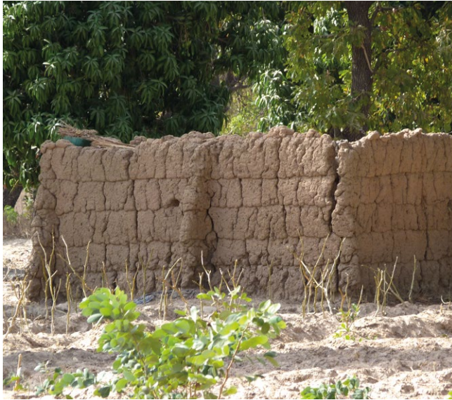
Wall with overlapping profiled courses and buttresses to provide stability in a Birifor construction.
