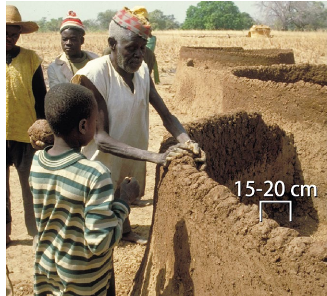
Construction of a cob wall.
