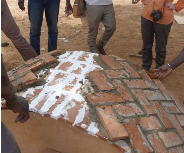
Execution of the second layer.
