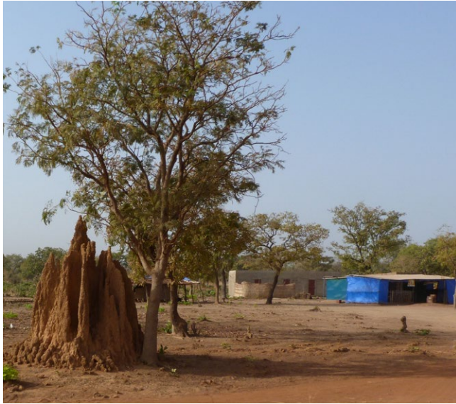
Aerial termite nest beside a tree and close to a house, a potential cause for issues in timber structures.
