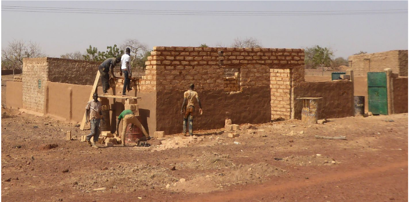
Construction of a dwelling with adobe.
