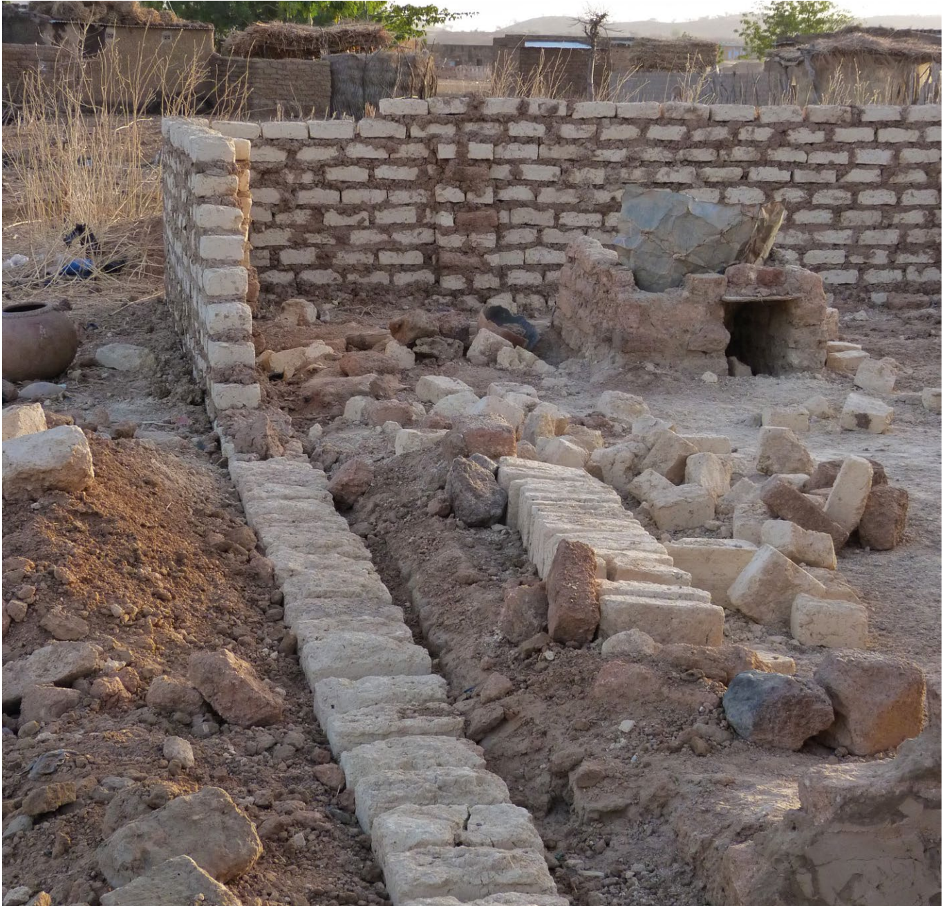
Adobe course used for foundations.
