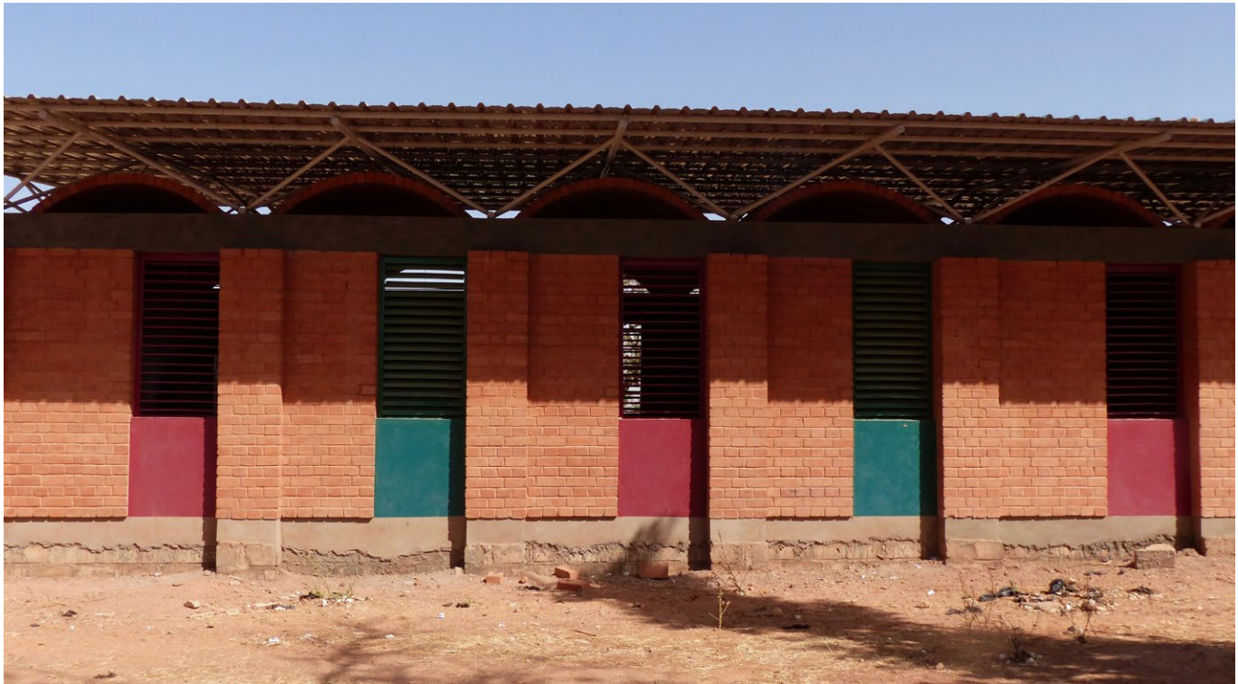
School classrooms, built during Phase 1 of the project, pending the basement of the building.
