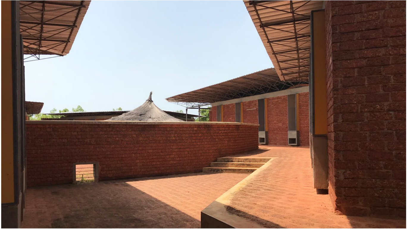
Noomdo Orphanage (Koudougou, Burkina Faso), designed by Francis Kéré.
