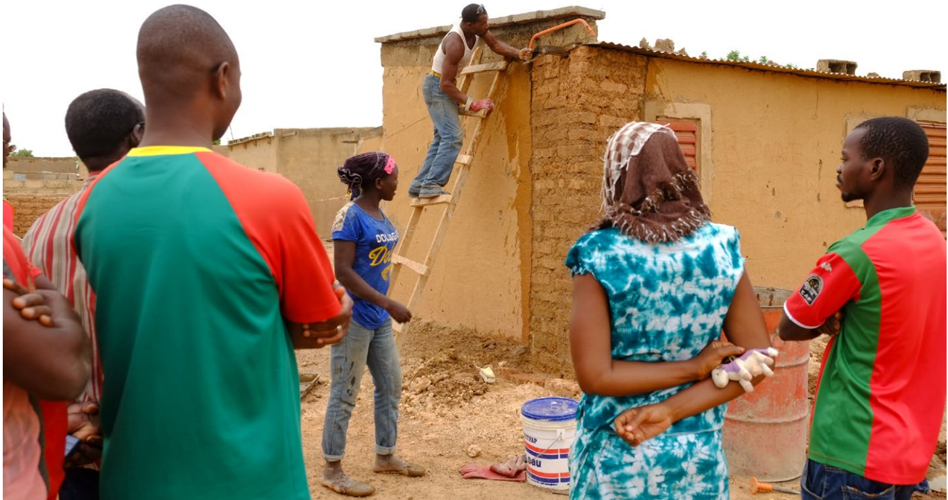
Repairing dwellings during the Boassa neighbourhood improvement project.
