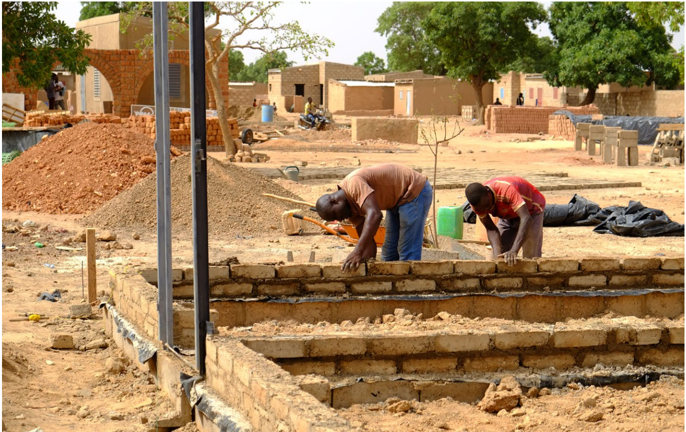
Construction of buildings during the Boassa neighbourhood improvement project.
