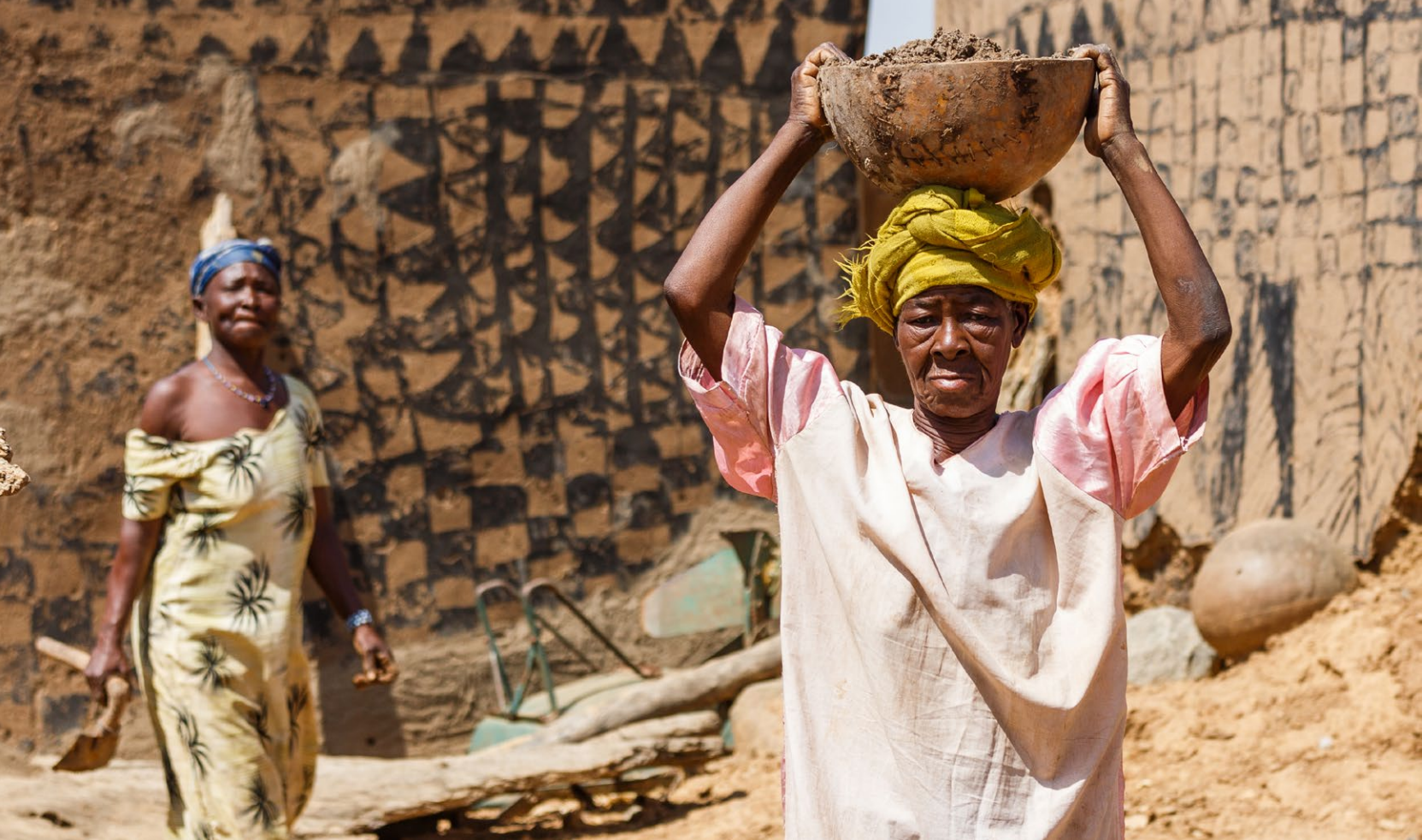
Kassena women transporting mud to carry out tasks for the maintenance, rendering and polychrome painting of the walls.
