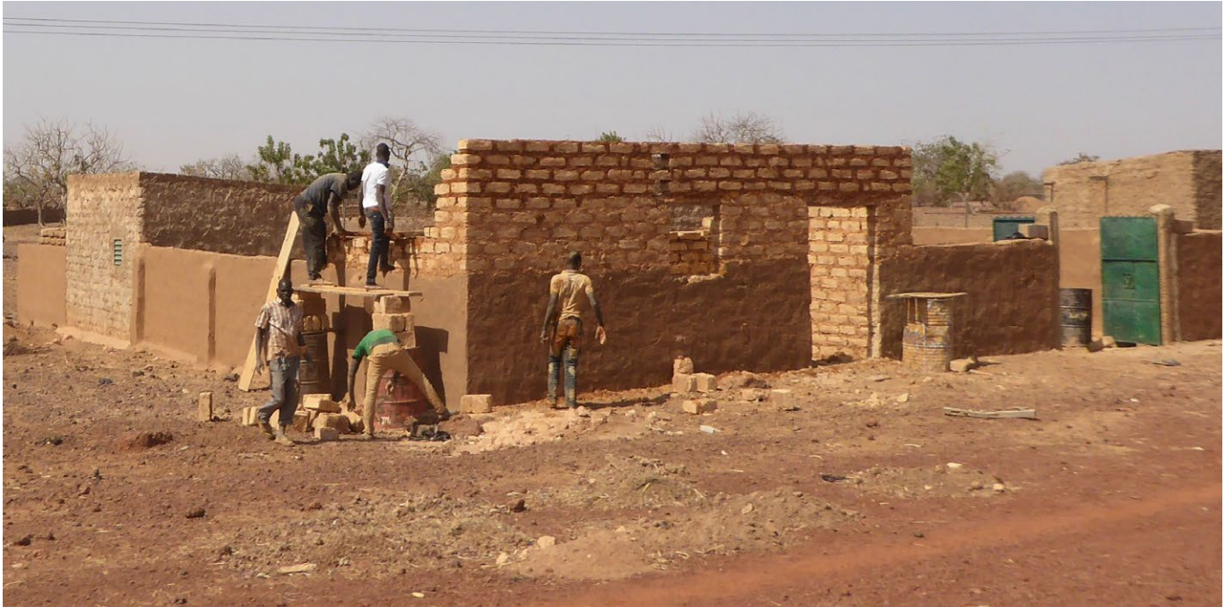
Construction of a dwelling with adobe.
