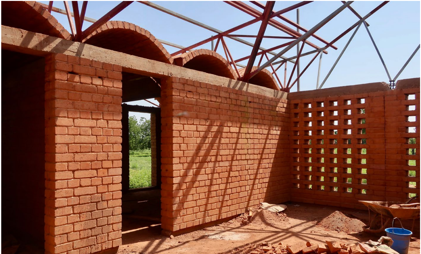
Interior of the administration building under construction, Phase 2 of the project.
