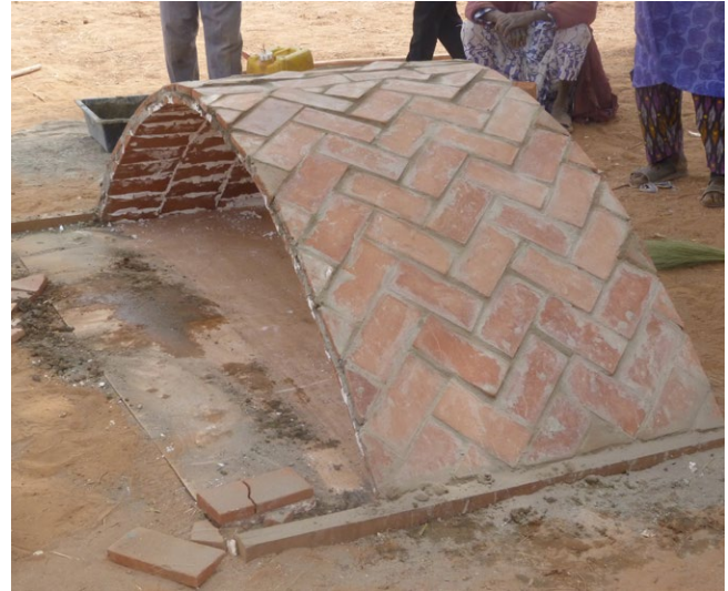
A finished vault in the Baasneere workshop.
