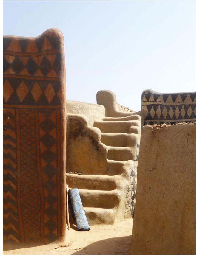
Interesting masonry stairs in a Kassena dwelling with an intermediate staggered separation between the first flight of steps, also used as seats, and the second, specifically for accessing the flat roof.
