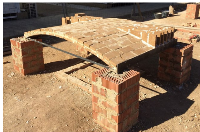
Complete CEB tile vault and tests for the construction of small wall partitions to support the paving.
