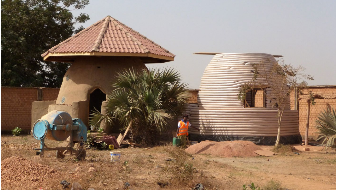
Earthbag construction domes in Ouagadougou.
