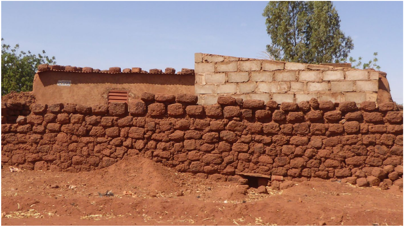
Wall in laterite masonry and wall in precast concrete blocks.
