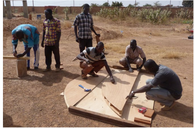
Construction of the wooden centring.
