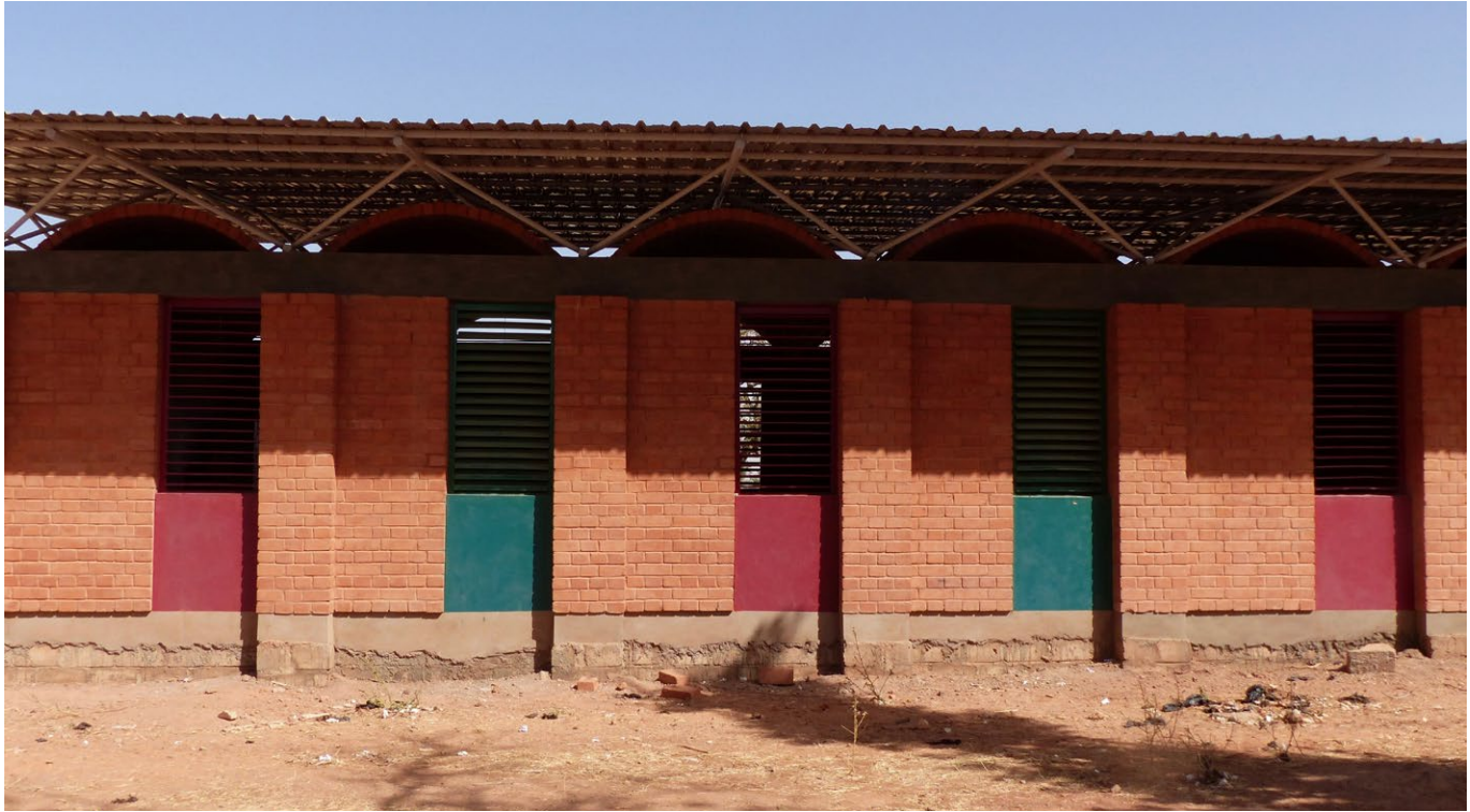
School classrooms, built during Phase 1 of the project, pending the basement of the building.
