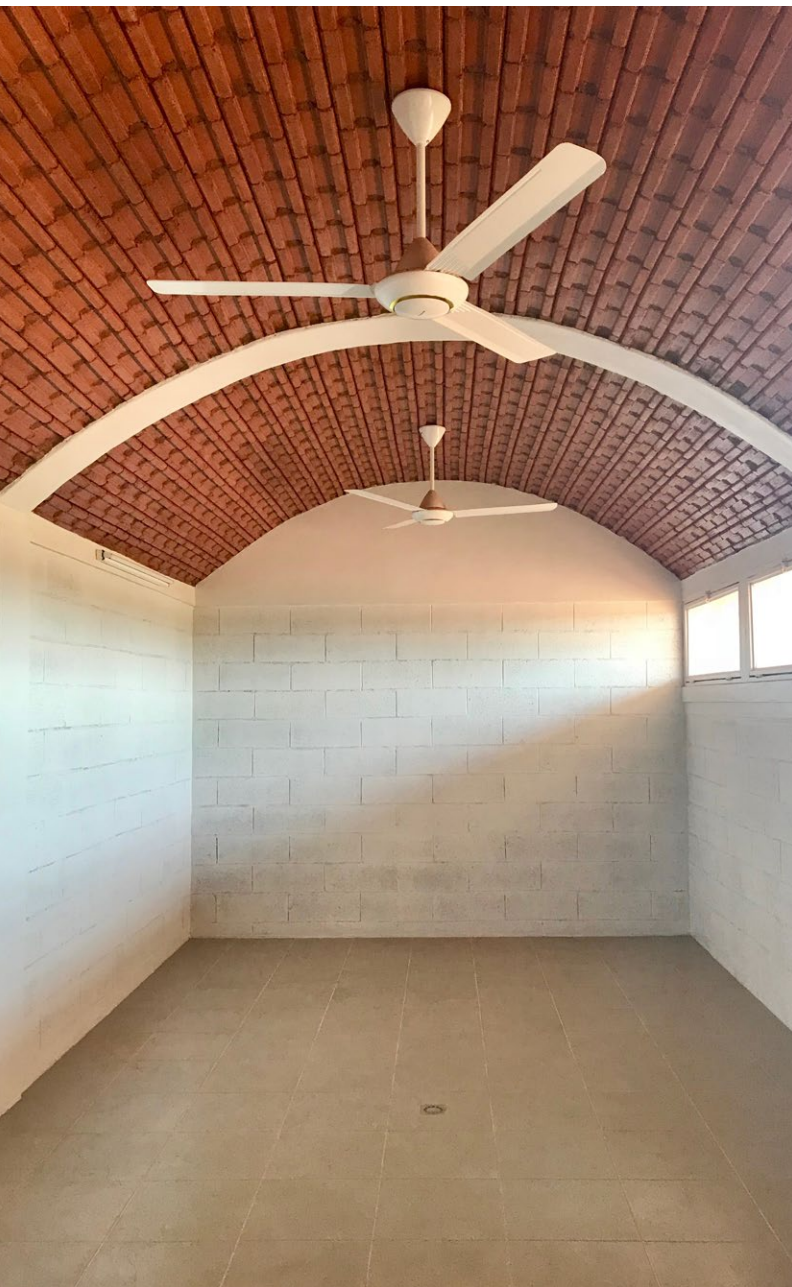
One of the rooms of the opthalmological block in Boulmiougou (Ouagadougou).
