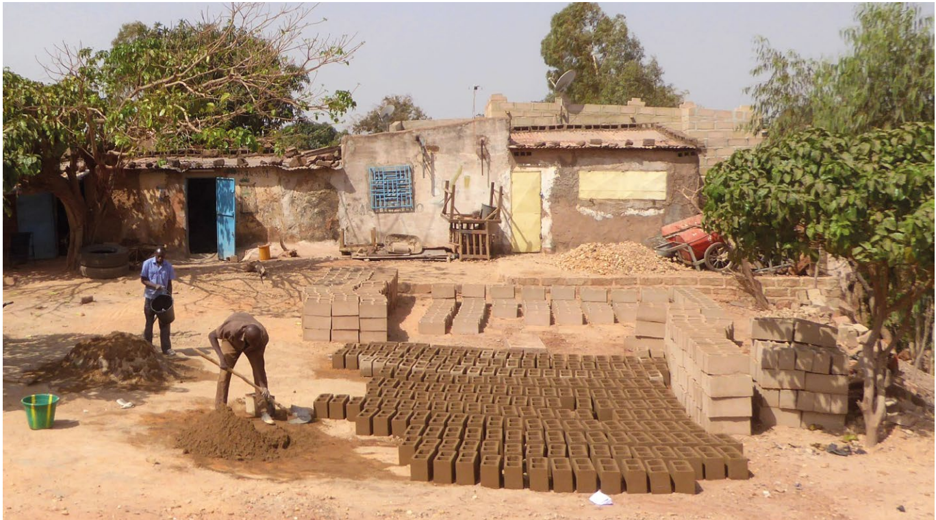
Current production of precast cement blocks in Banfora.
