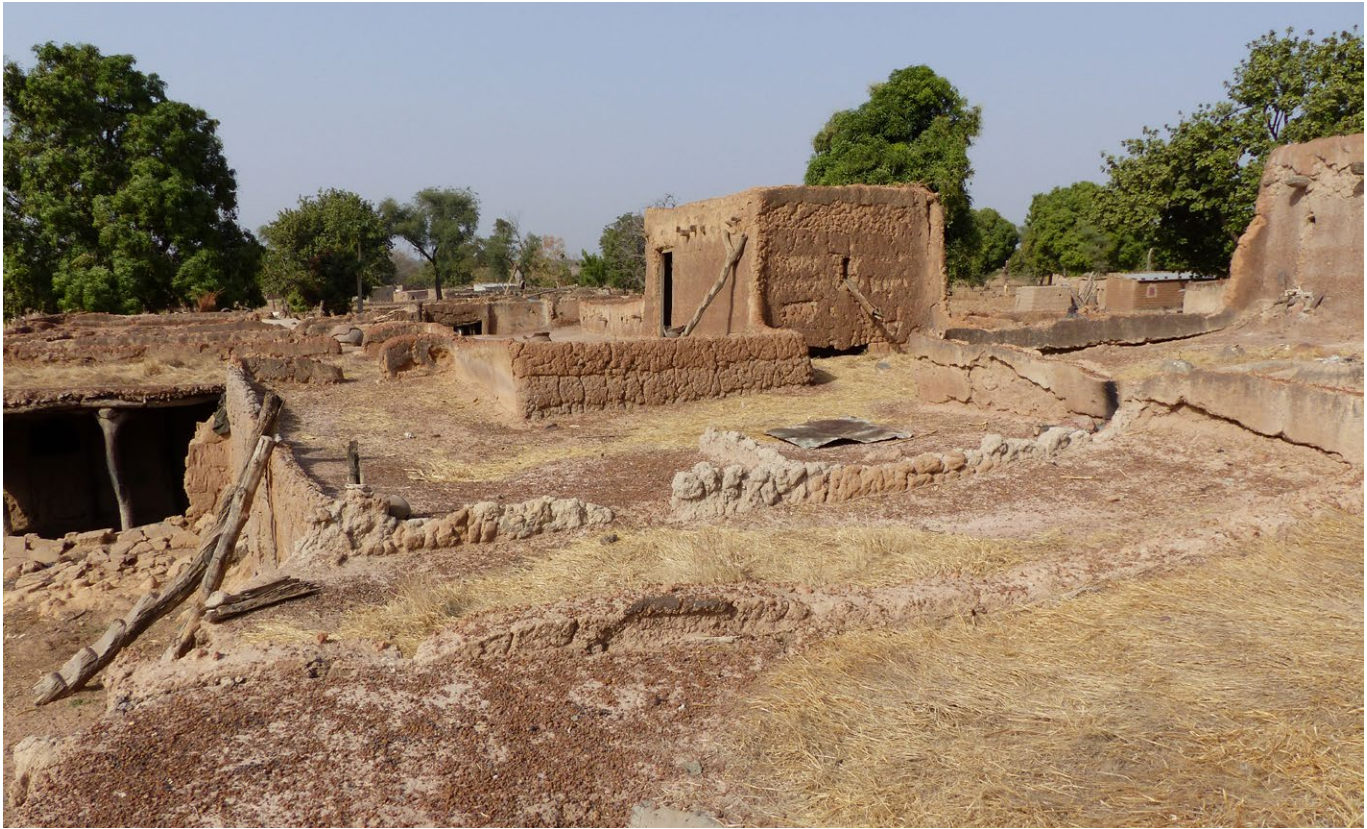
The Birifor flat roof, where all sorts of activities are carried out, becomes the extension of the dwelling itself.
