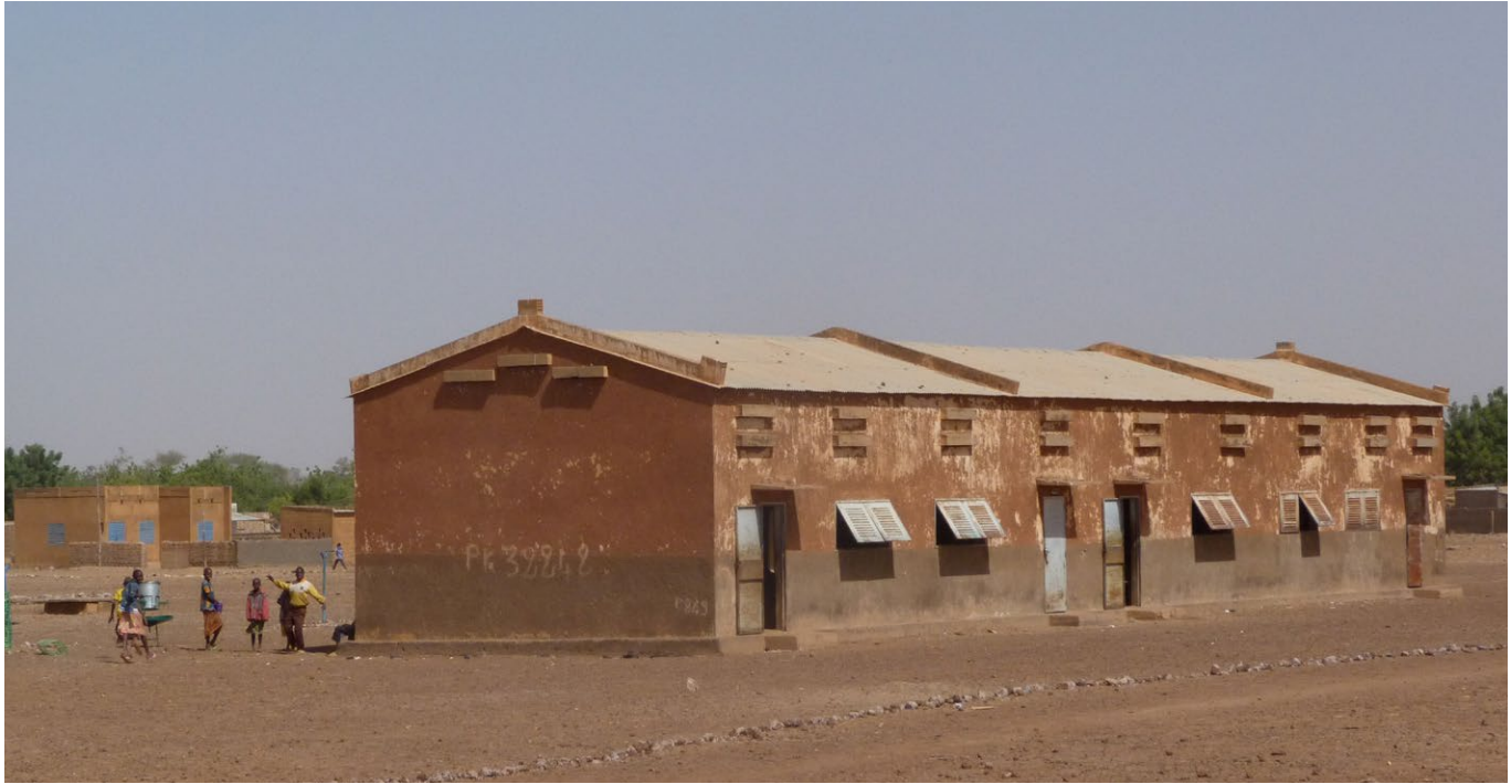
A conventional school built with concrete blocks and sheet metal. Baasneere, Burkina Faso.
