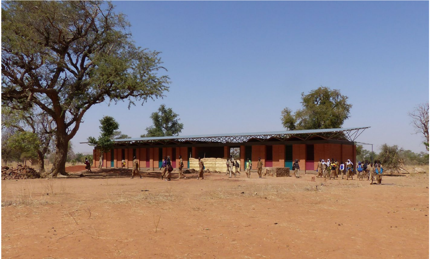
School classrooms, built during Phase 1 of the project.
