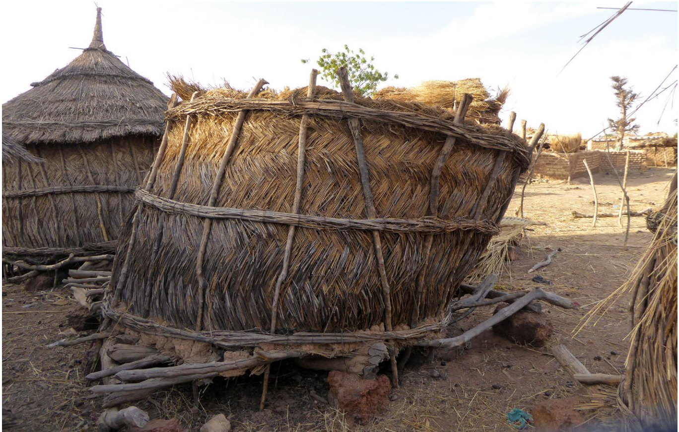
Mossi silo with plant walls which have lost their form as their creeper hoops have loosened and the perimeter palisade has moved.
