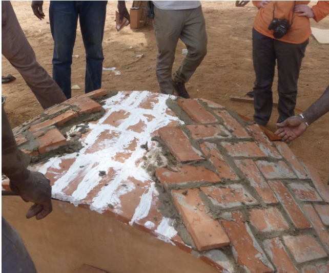
Execution of the second layer.
