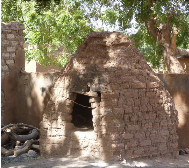
Bread oven with a pointed domical vault truncated at the top.
