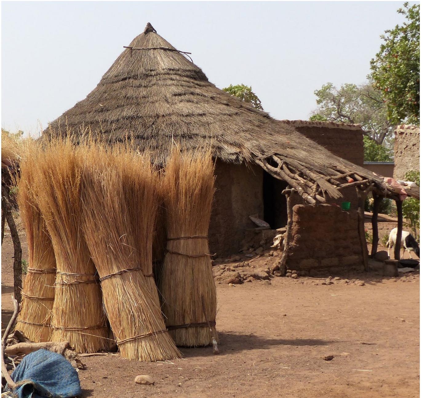
Bundles of straw prepared to repair existing roofs in a Gan village.
