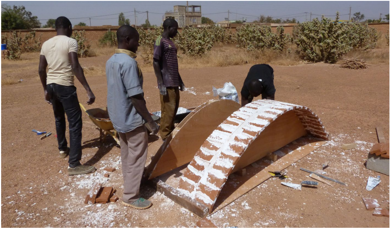
Construction of the inner layer of the vault.
