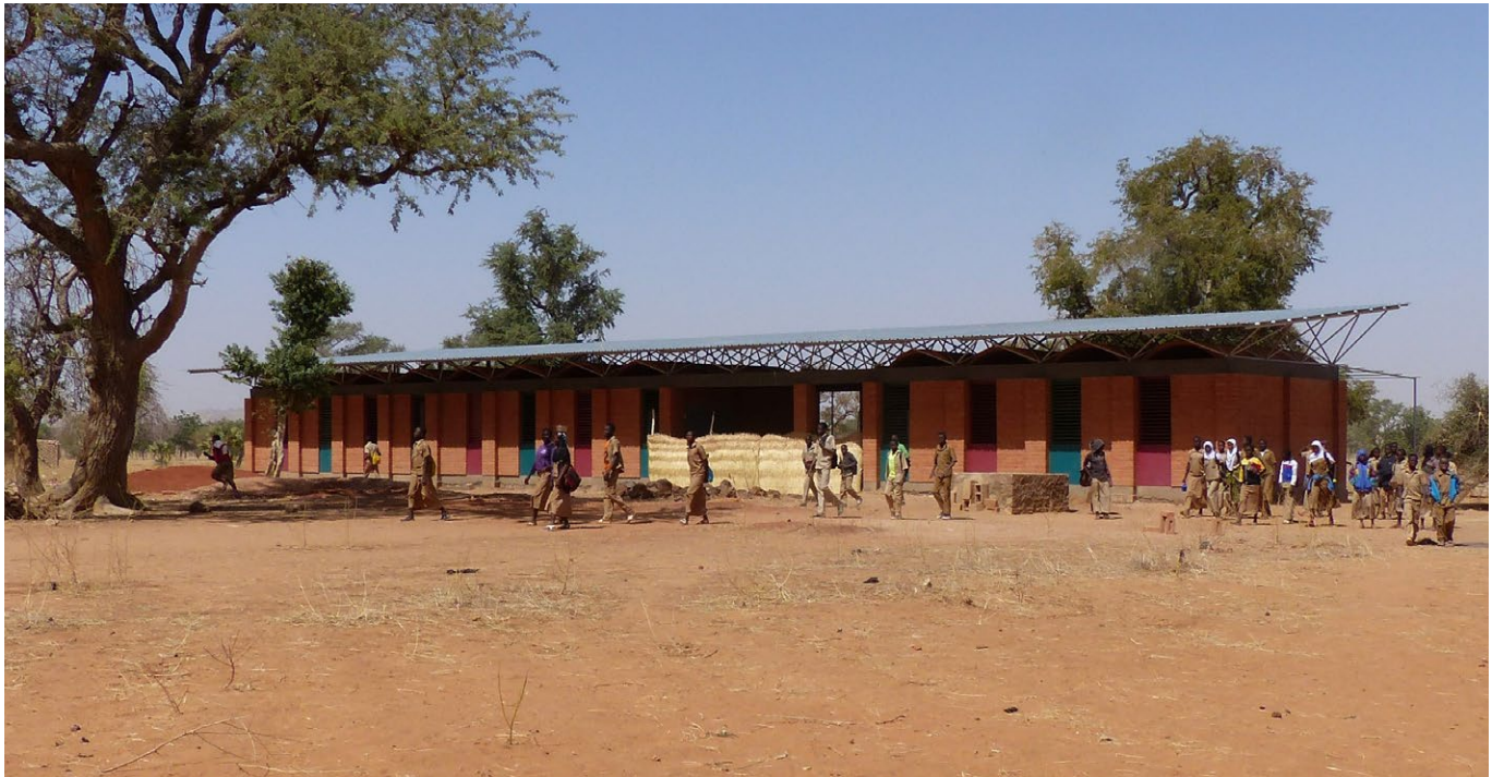
Classroom building for the secondary school developed by Algemesi Solidari.
