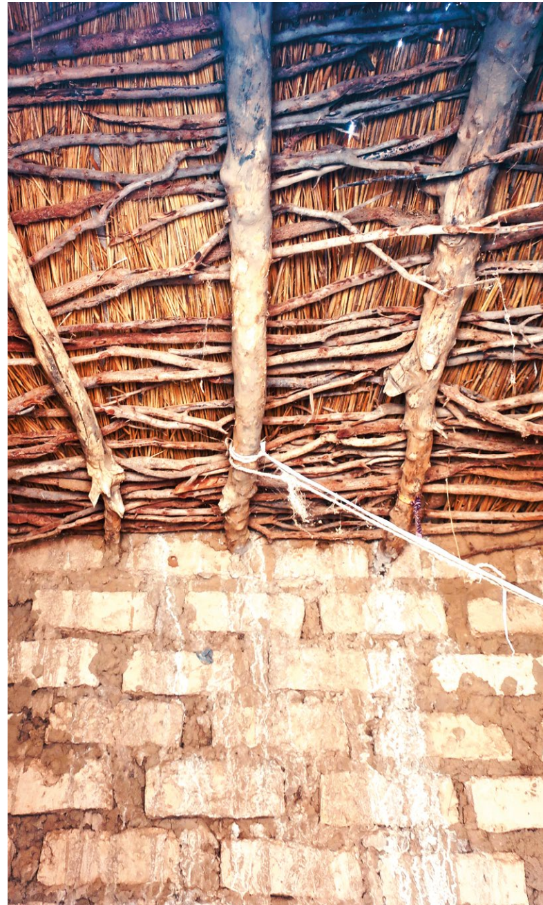
Inner view of a traditional roof.
