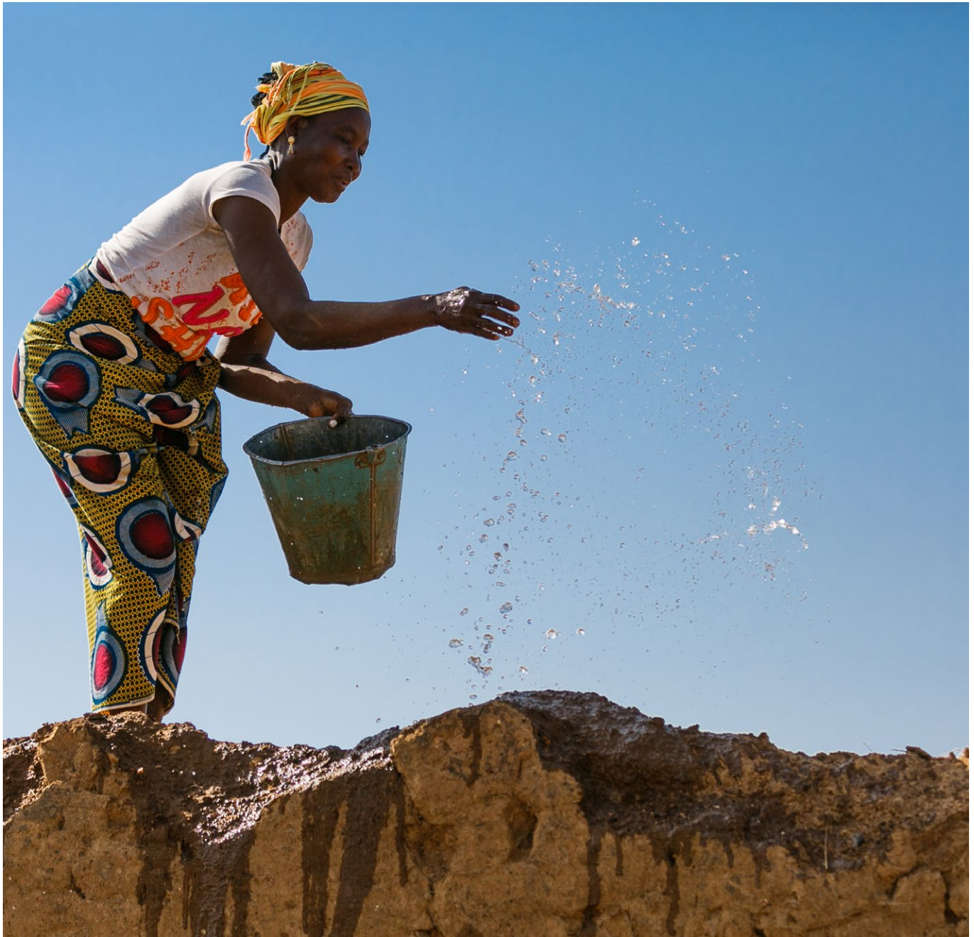
Kassena woman sprinkling water on the flat roof prior to repair.
