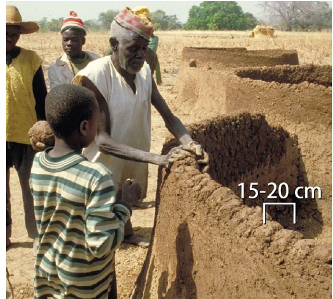
Construction of a cob wall.
