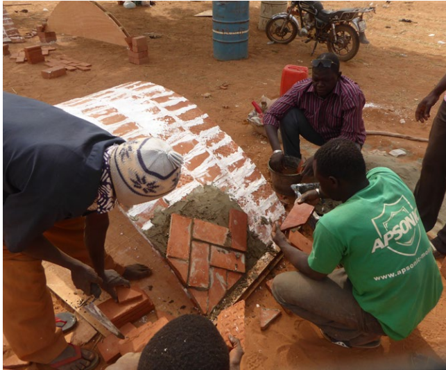
Vault construction workshop in the village of Baasneere.
