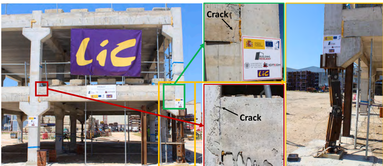
Fig. 25. Structure after the test.
