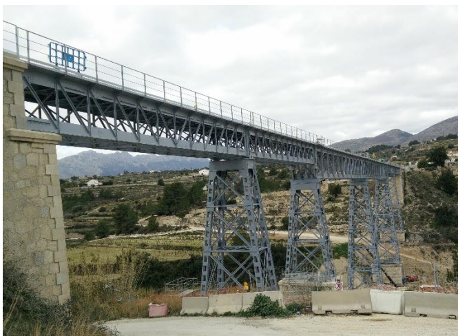
Figure 3. Real case study. Quisi bridge (Valencia, Spain). General view
