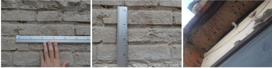
Fig. 16 Dimensions of the brick units and thickness of the façade. (Source: Authors 2022)
