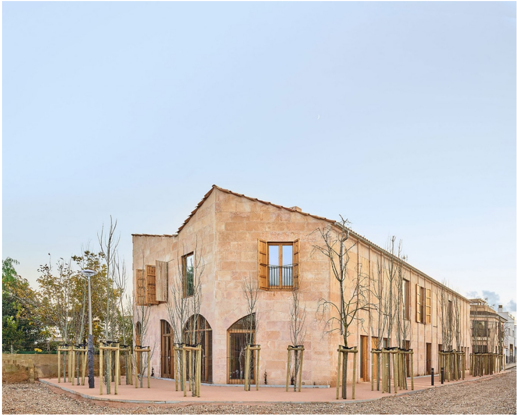
Figure 3. IBAVI, Social Housing in Palma de Mallorca, 2021. Outside view. (Credit: José Hevia)
