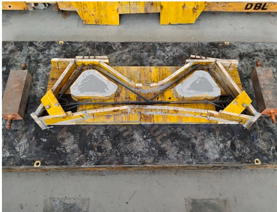
Fig. 16. Casting of the deviator. Left: formwork and minimum reinforcement; right: the deviator after unmoulding.
