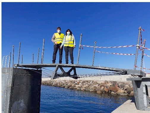
Fig. 21. The footbridge in the final location. The image on the right shows the finished cable handrails as well as a non-structural lateral baseboards. The cable anchored to the wharf at the forefront is securing the block on the water and is not attached to the footbridge.
