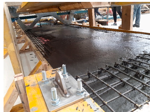
Fig. 17. Casting of the deck. Upper-left: formwork table and prestressing tendons and devices; upper- right: countermould prepared above the formwork and positioned deviator; lower row: two images of the casting process.
