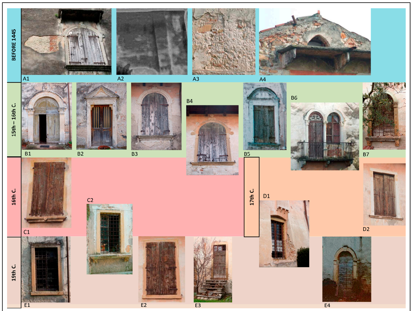
Figure 6. Abacus representation of exterior doors and windows of the building in chronological order. The openings have been grouped into four chronological phases (represented by the colored stripes) and have been named with a capital letter corresponding to the period and an identification number.
