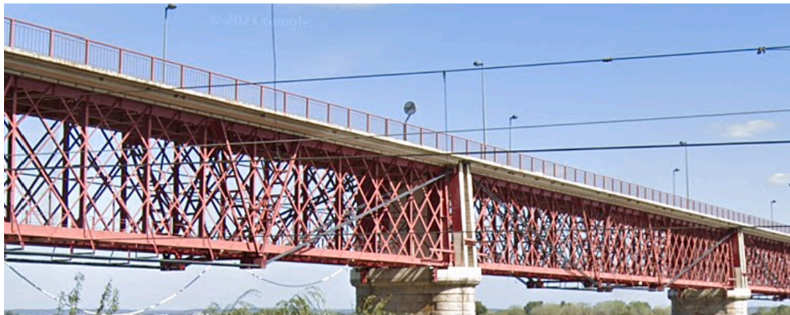
Fig. 2. Truss bridge studied.
