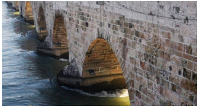
Figure 14. Eddy caused by increase in the average velocity in the levees.
