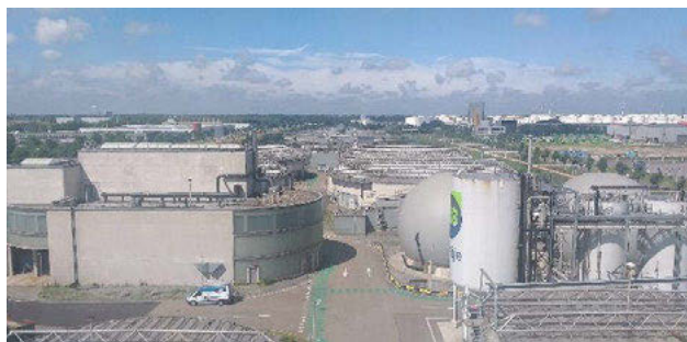
Figure 1: Amsterdam West WWTP
