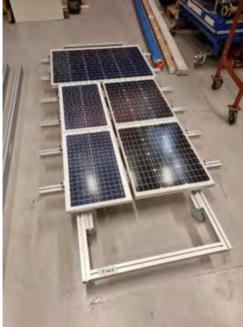
Figure 73. PV Panels Installation on the Support Structure.
