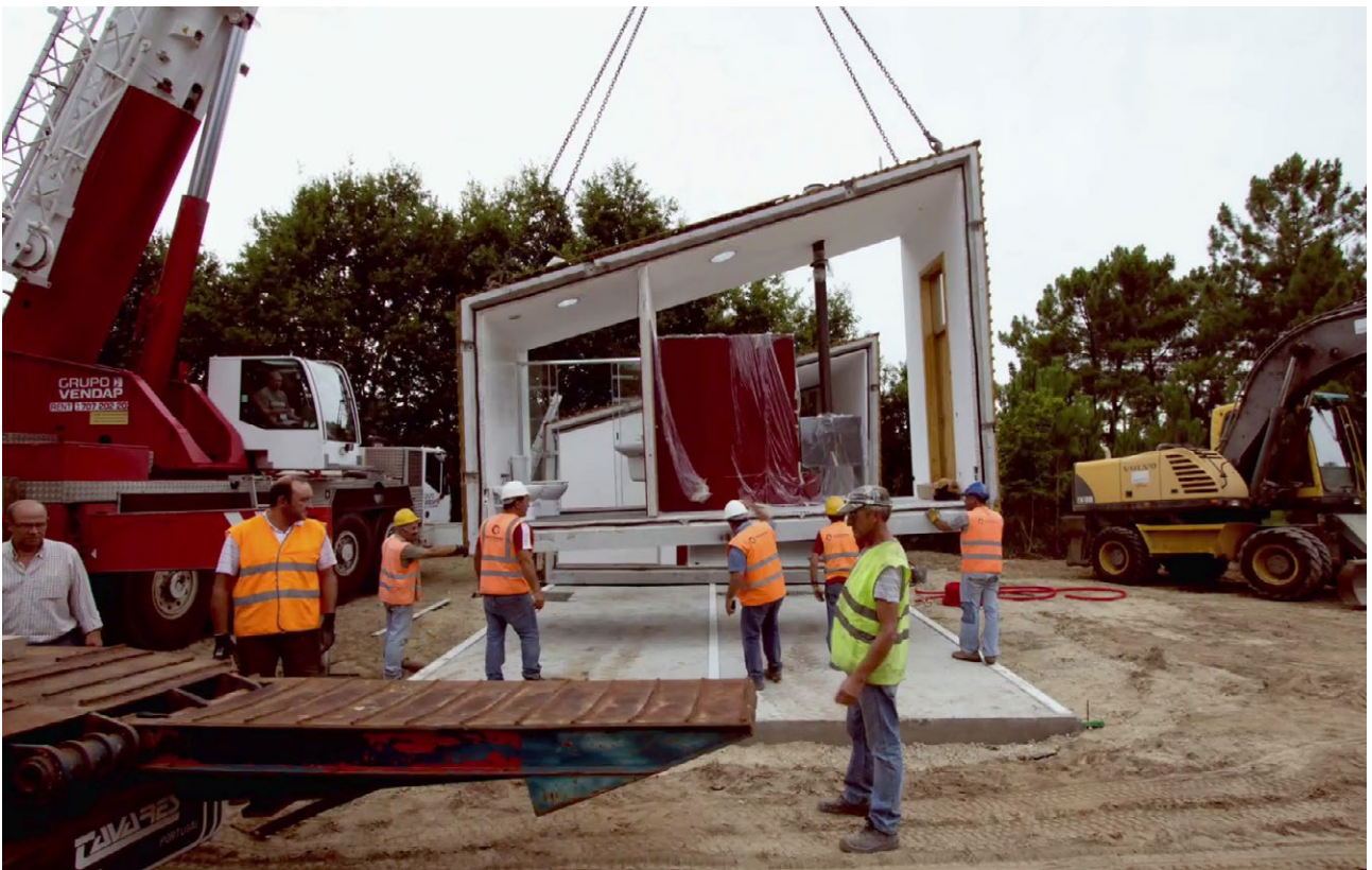
Figure 3 | On-site handling of the module, video still, credits: Building Pictures.
