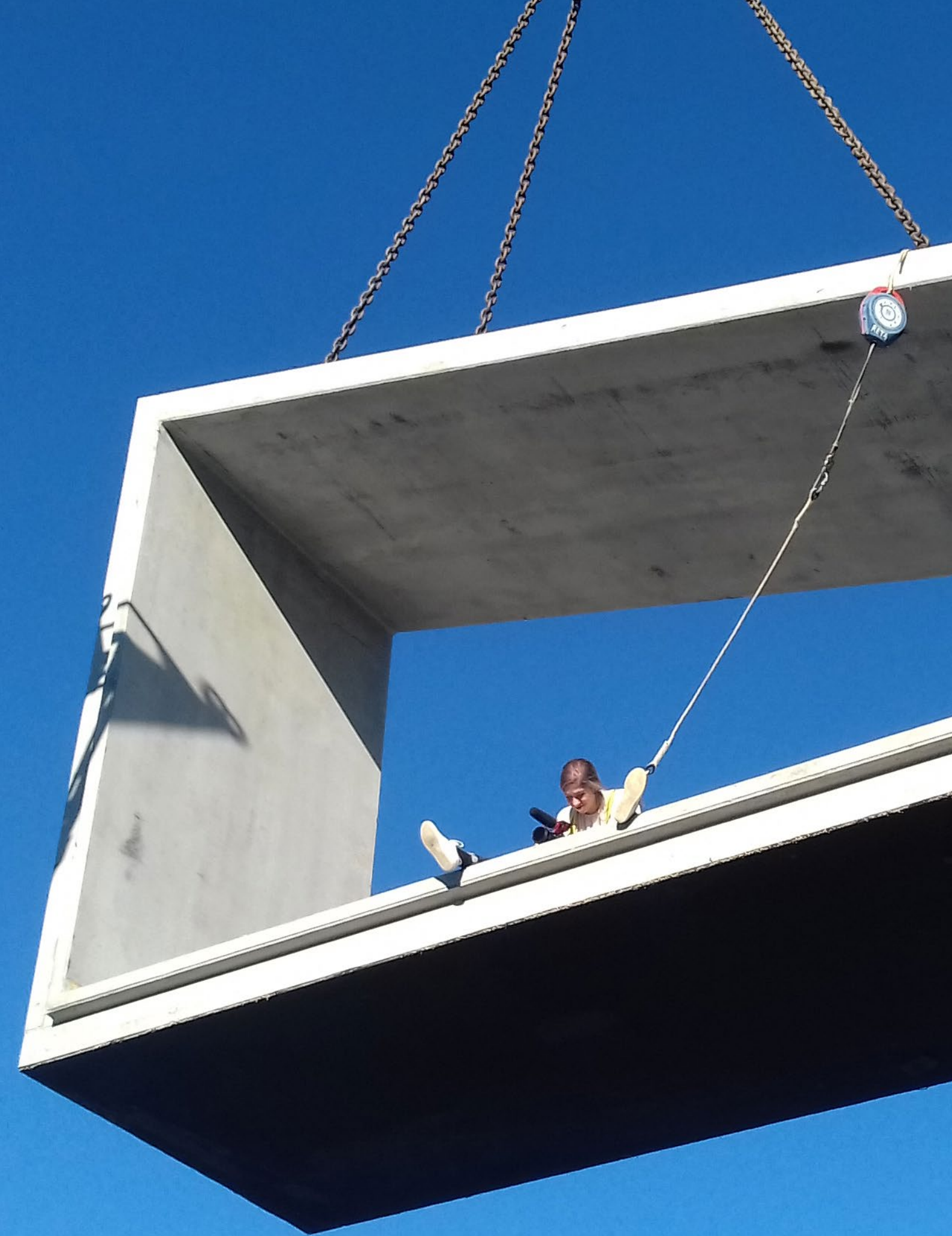
Gomos modular system, Vale de Cambra, Portugal, photo by Building Pictures.
