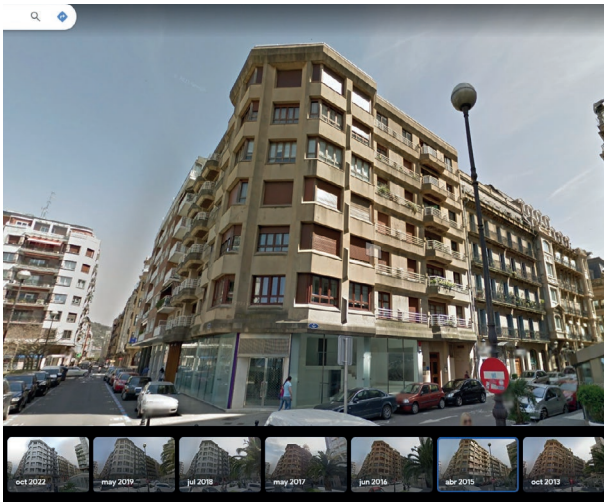
Fig. 1. Image of the building at Calle Triunfo 1. 2023 (Source: Google Maps, 2015).
