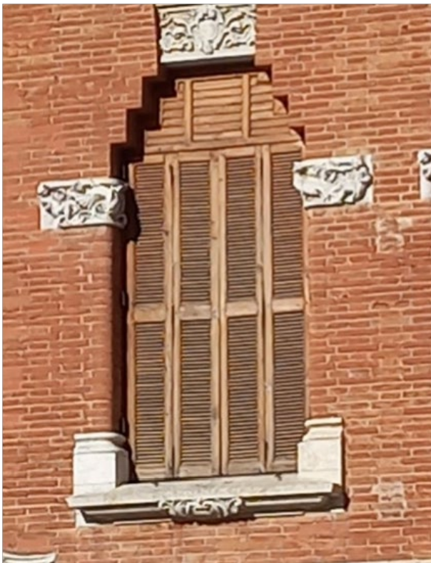
Fig. 7. Above: Facade. Below: Details where the combination of materials can be seen: brick, stone and ceramic.
