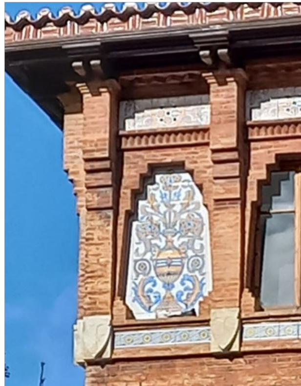
Fig. 7. Above: Facade. Below: Details where the combination of materials can be seen: brick, stone and ceramic.
