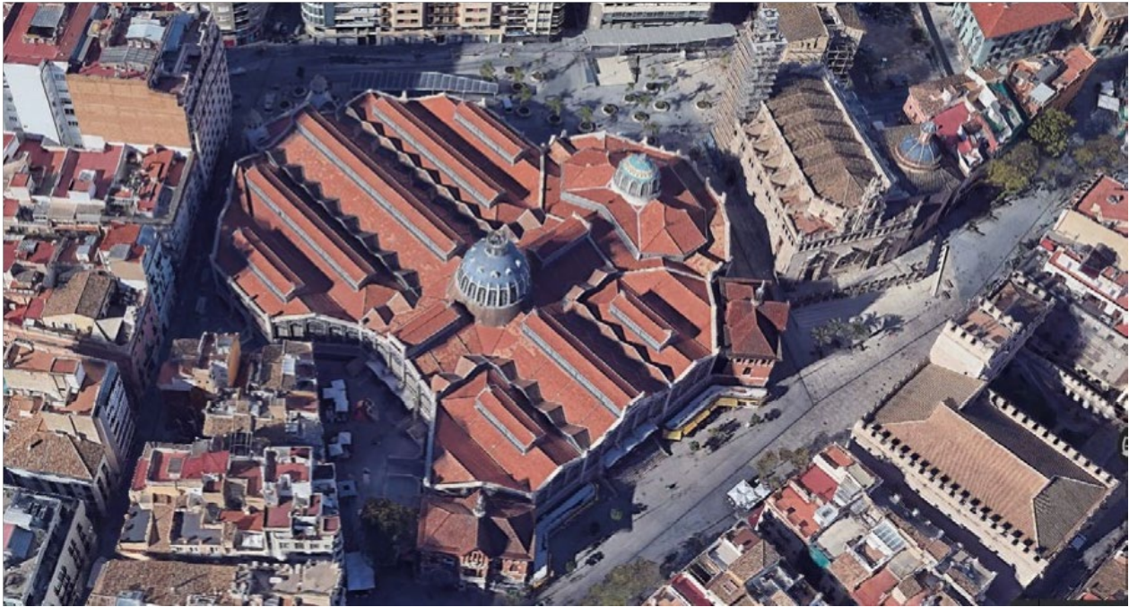
Fig. 2. Aerial view of the Central Market. The two orthogonal axes with a dome above the transept can be seen. The plant adapts organically to the sun.
