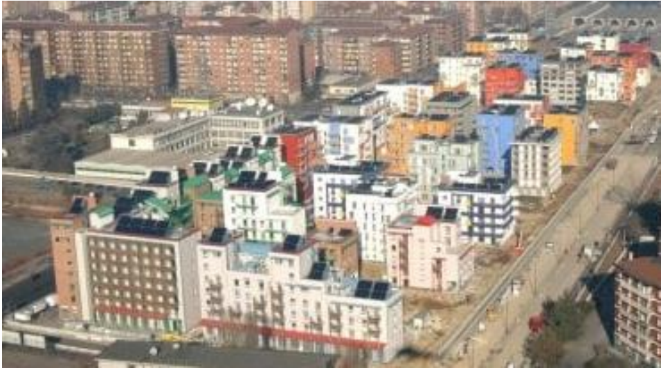
Figure 37 Picture showing the Olympic village – view 01 49
