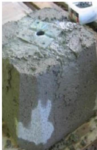
Figure 268 Picture showing support positioning after cement fill 287
