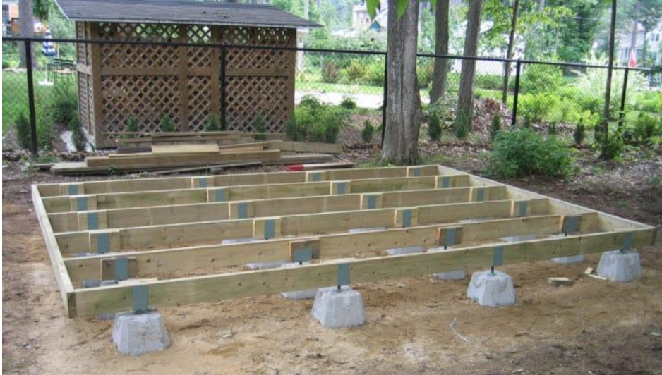
Figure 269 Picture showing timber beams positioned into the brackets 288
