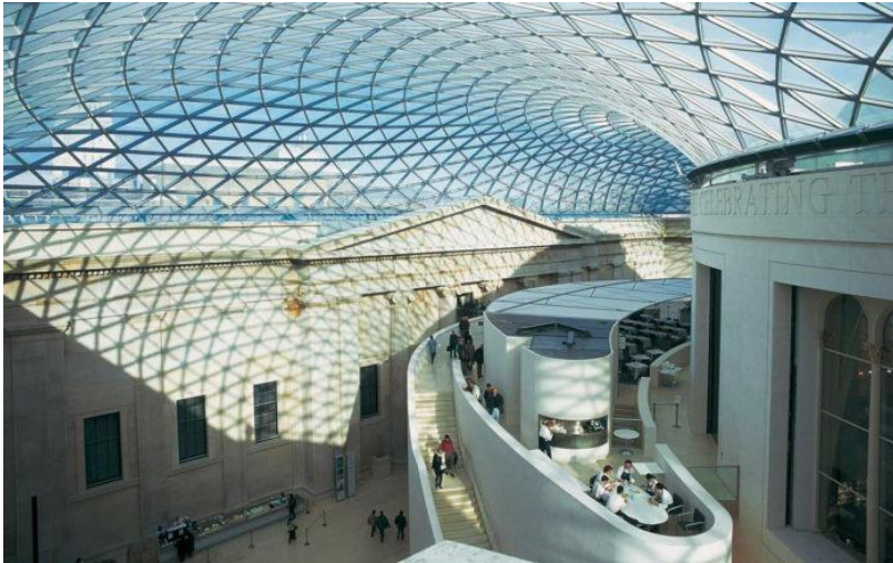
Figure 45 Picture showing the steel skylight of the Museum 59
