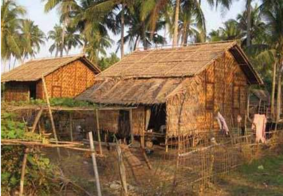
Figure 189 Picture showing the Twin elevated shelter unit 206
