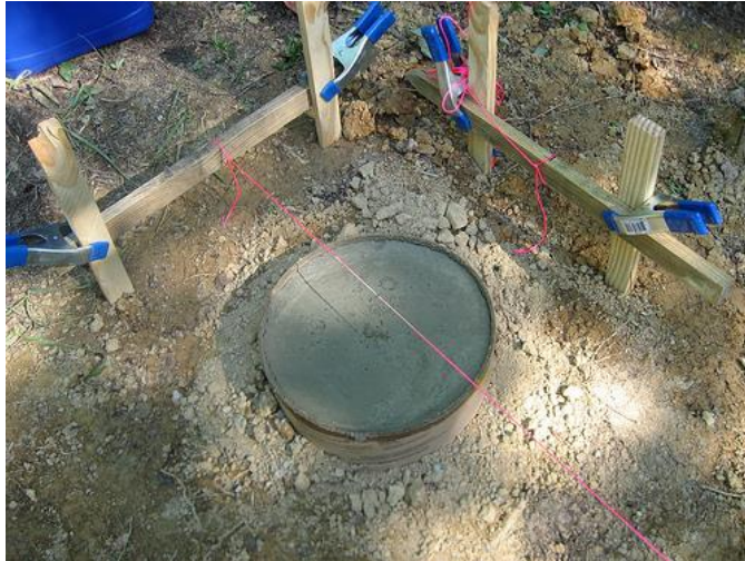
Figure 281 Picture showing filled concrete tube forms 300
