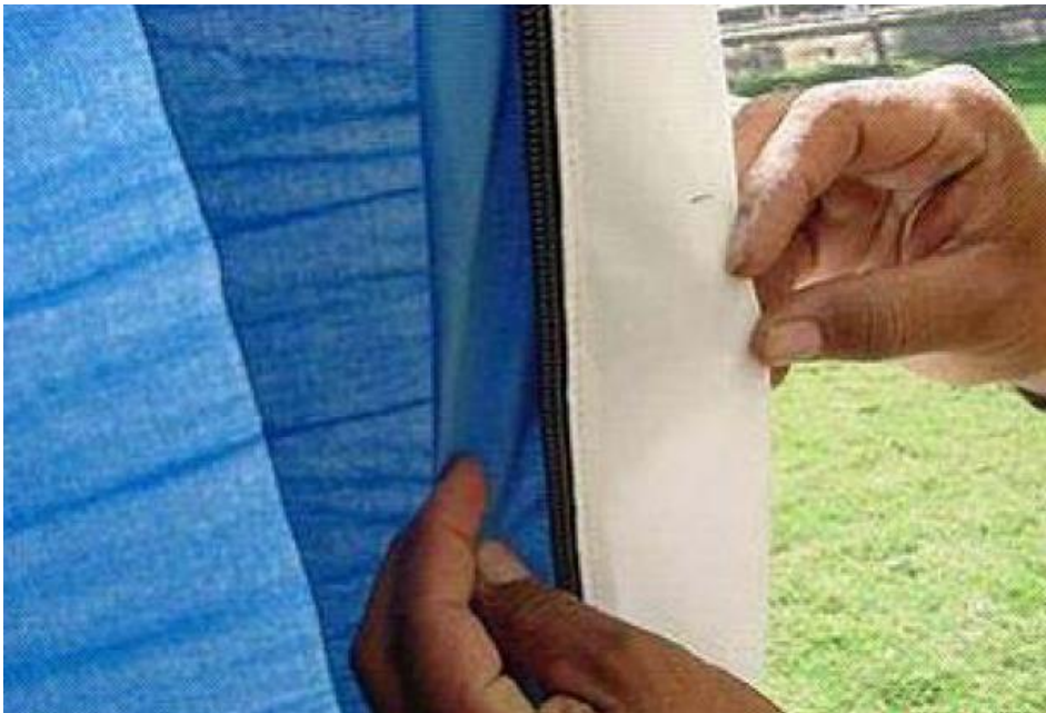
Figure 364 Picture showing the zipper and the double folded door of an UNHCR tent-1 305
