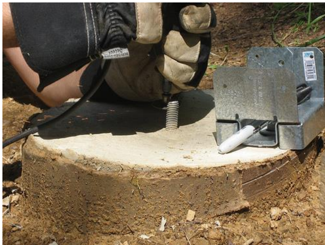
Figure 282 Picture showing the steel post anchor bolt 301
