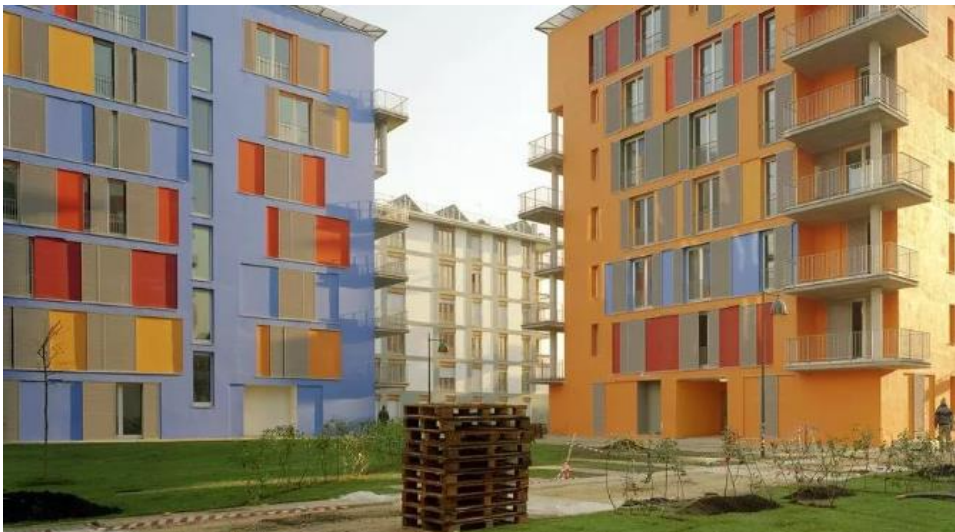
Figure 38 Picture showing the Olympic village – view 02 50
