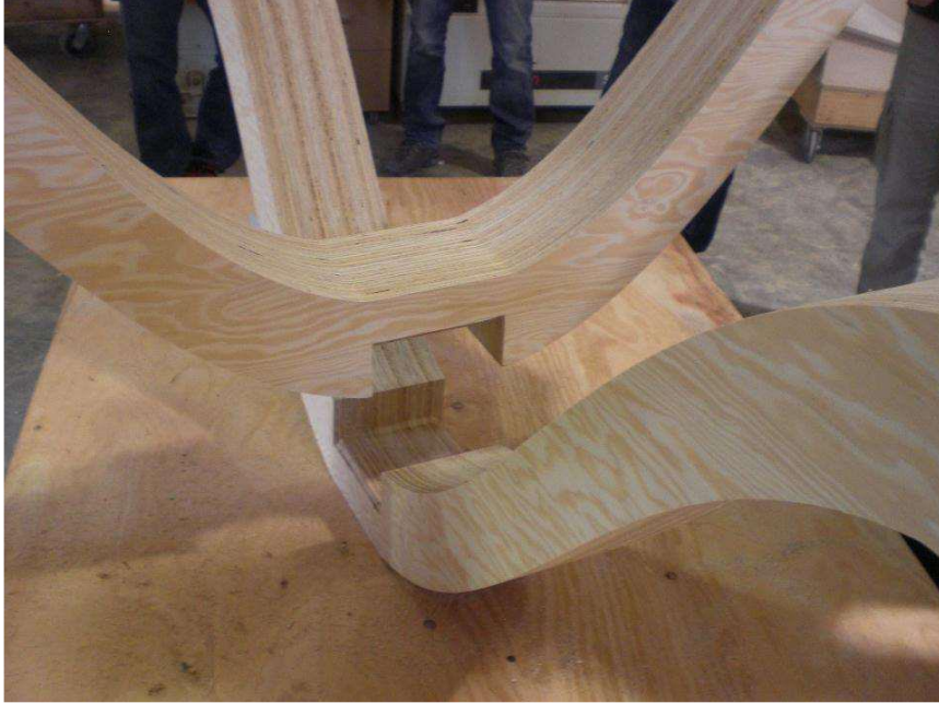
Figure 146 Picture showing the space frame web connection 163
