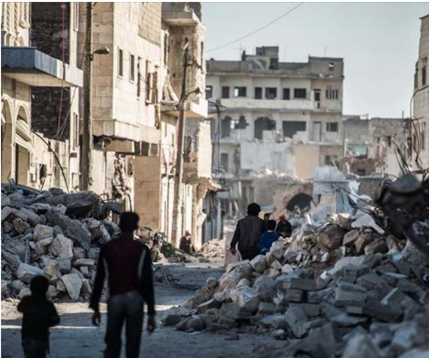
Figure 20 Picture showing the level of destruction due to the civil war 26
