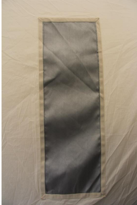
Figure 373 Picture showing a typical chimney reinforcement designated area in a UNHCR tent. 306
