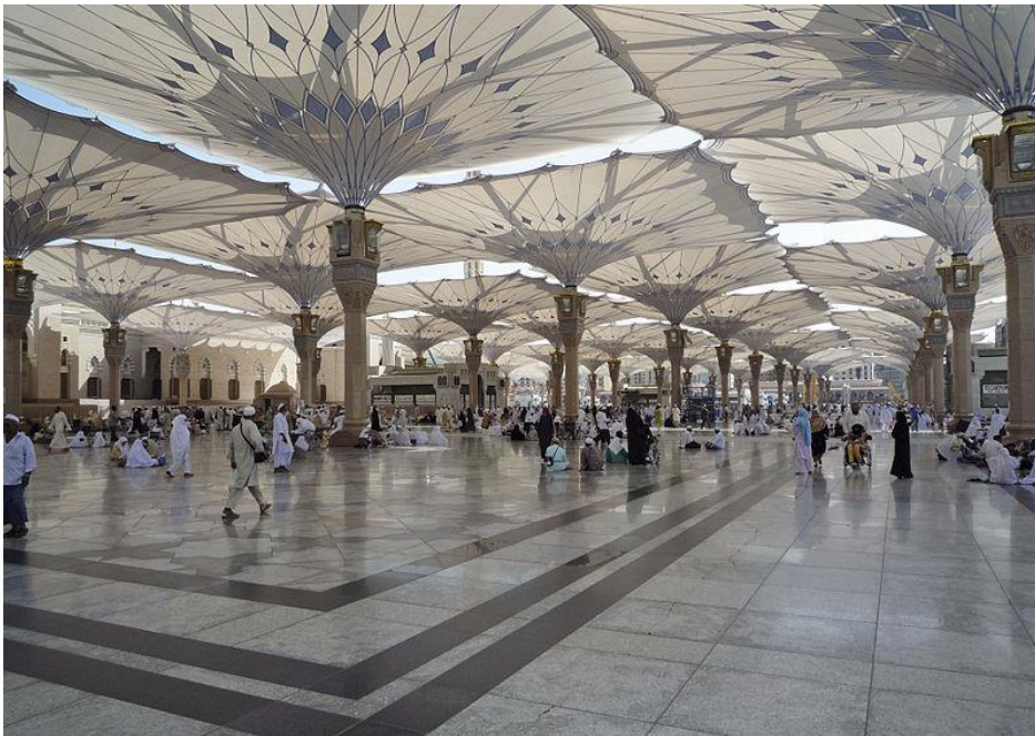
Figure 157 Picture showing architect Mahmoud Bodo Rasch's convertible shading tensile structure 174
