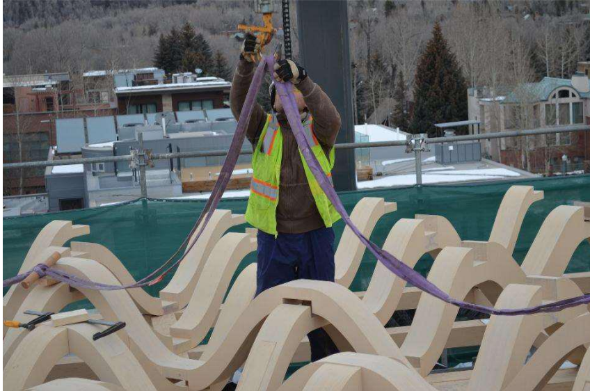
Figure 150 Picture showing fitting between layers was not always smooth 167
