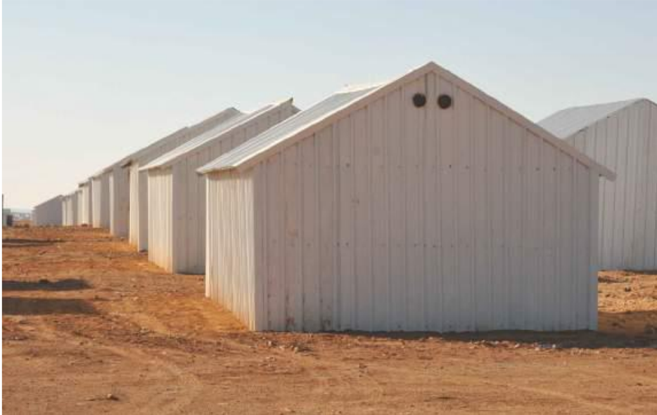
Figure 185 Picture showing the T-shelter unit 202
