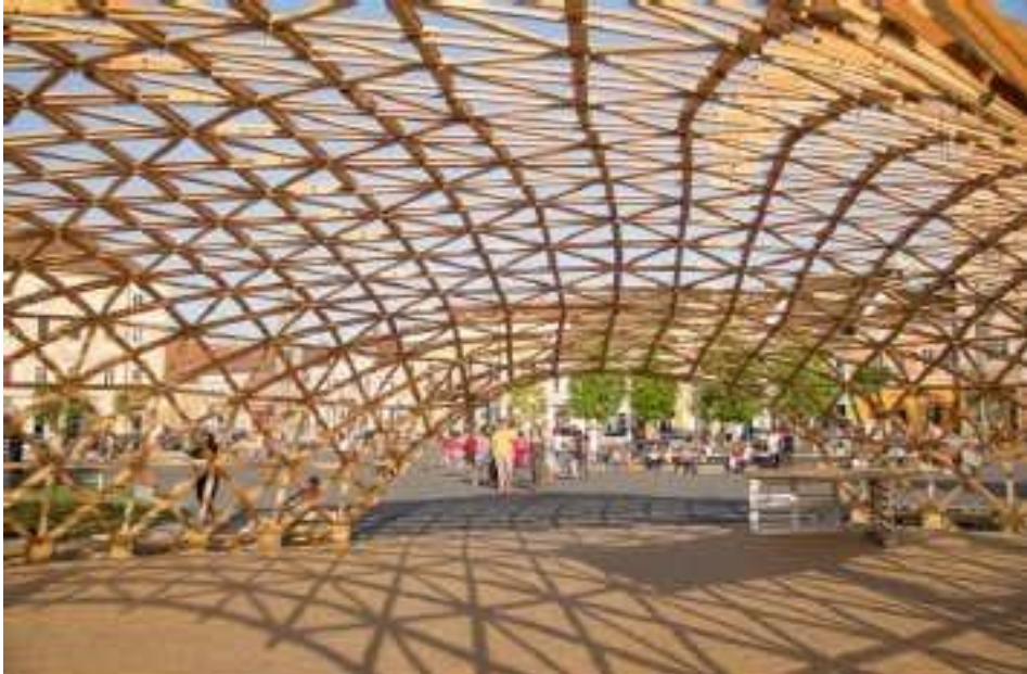
Figure 61 Picture showing the interior of the Pavilion ZA Gridshell 75
