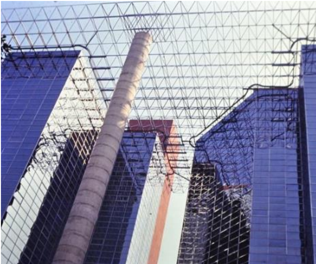
Figure 76 Picture showing a flat cover structure 90
