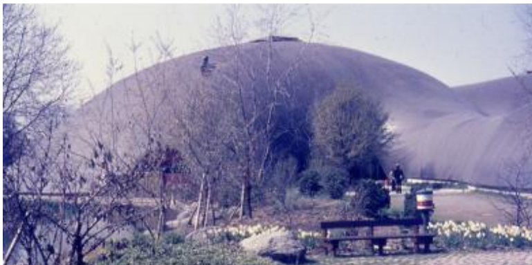
Figure 72 Picture showing the PVC translucent covering 86
