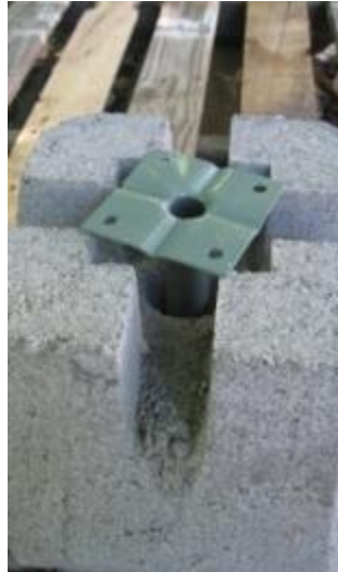
Figure 267 Picture showing support proper edge positioning 286
