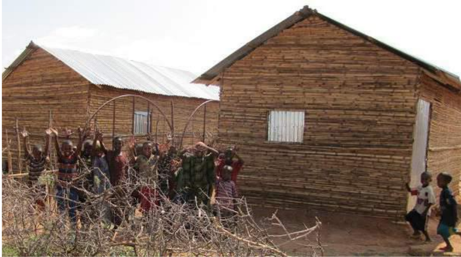
Figure 187 Picture showing the Compact Bamboo shelter unit 204
