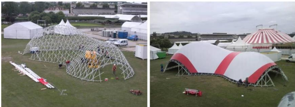
Figure 48 Pictures showing Gridshell in composite materials for Solidays festival in Paris 62
