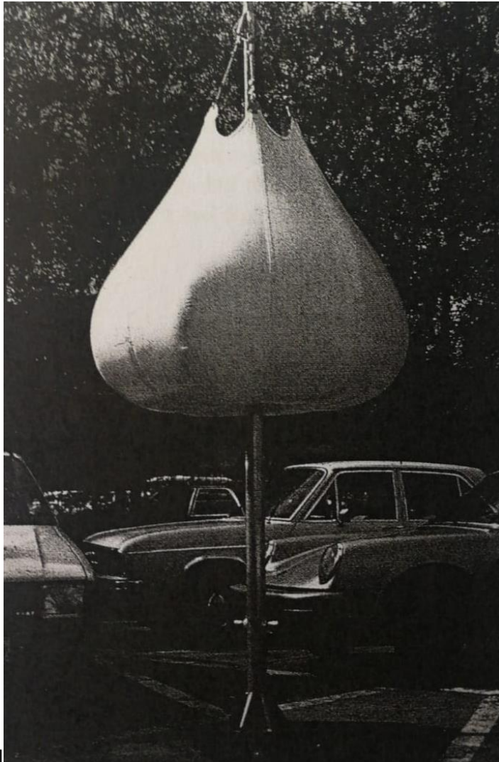
Figure 162 Picture showing an air supported Synclastic structure 179
