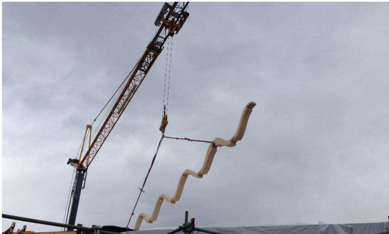
Figure 149 Picture showing crane being used for heavy lifting 166
