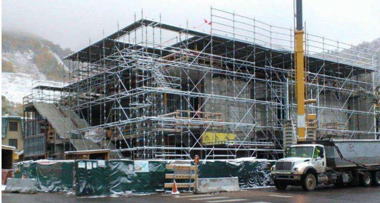
Figure 148 Picture showing scaffolding 165
