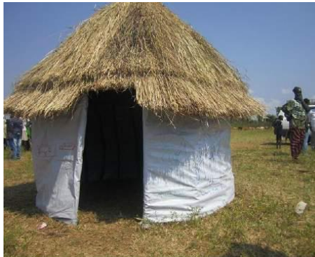
Figure 182 Picture showing the shelter unit 199
