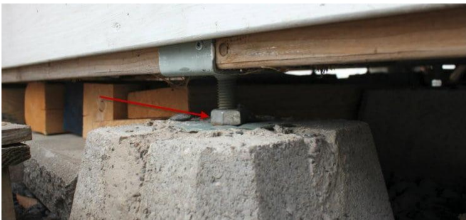
Figure 270 Picture showing nut used for level adjustment 289
