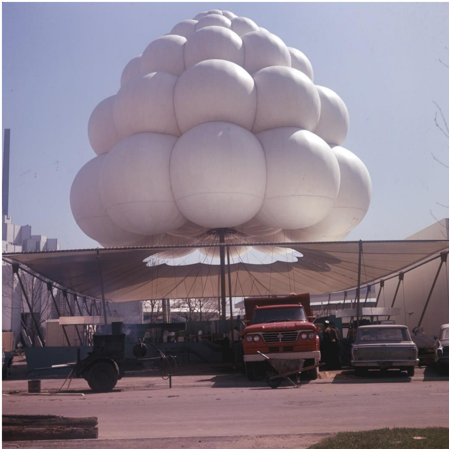
Figure 160 Picture showing an air supported Synclastic structure 177
