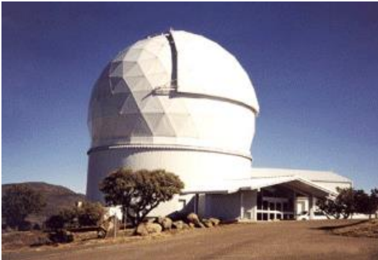
Figure 78 Picture showing a spherical dome structure 92
