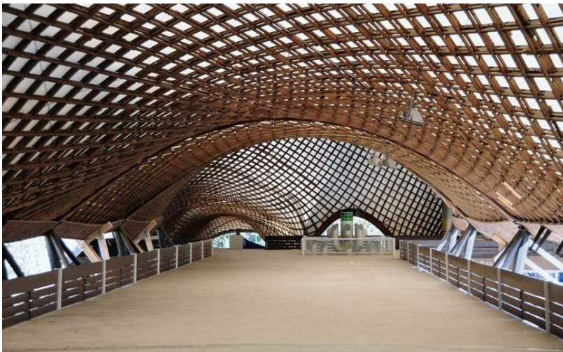
Figure 46 Picture showing the interior of the Mannheim Multihalle 60
