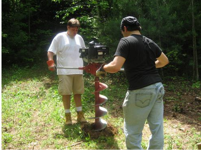
Figure 279 Picture showing the auger used for drilling the post anchor holes 298
