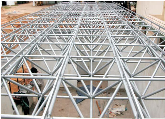
Figure 80 Picture showing a double layer space frame structure 94
