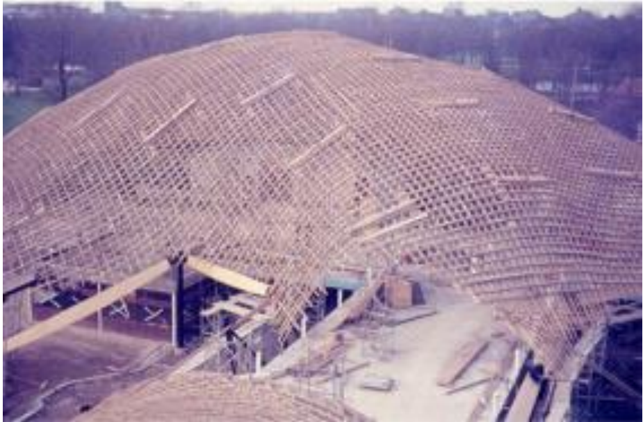
Figure 71 Picture showing the lifting arrangements on site 85
