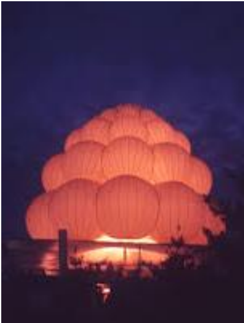
Figure 159 Picture showing synclastic structure of Walter Bird's Exhibition pavilion at the 1964 World Fair New York 176
