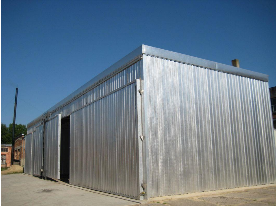
Figure 220 Picture showing an aluminum wood drying kiln 237
