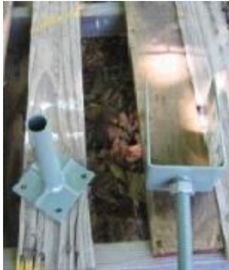
Figure 265 Picture showing separated base 284
