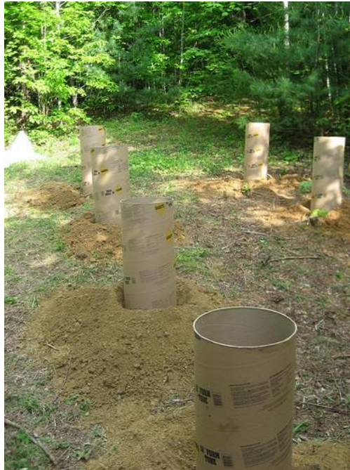
Figure 280 Picture showing concrete tube forms 299
