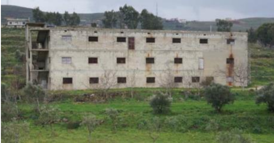
Figure 25 Picture showing a typical old abandoned building used by Syrian refugees 31
