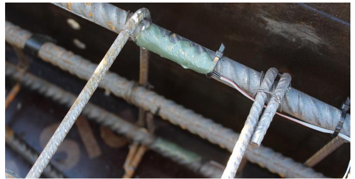
Figure 2. Strain gauge placed on main reinforcement of column prior to concreting.
