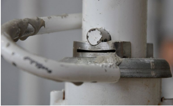
Figure 2. Structural fuse used to limit the maximum load a prop can bear.
