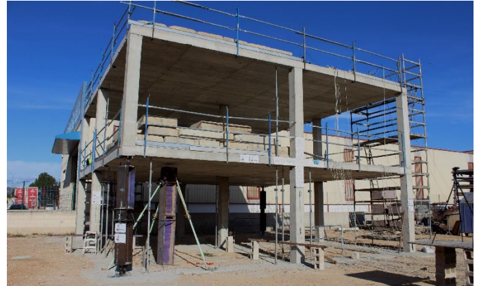
Figure 4. Test building prepared for sudden column removal.
