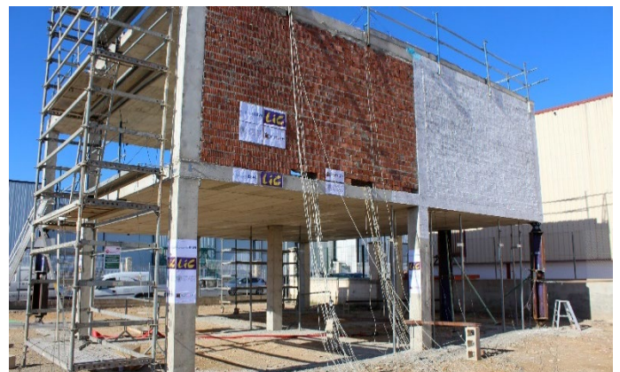
Figure 5. Test building for analysing the contribution of masonry infill walls.
