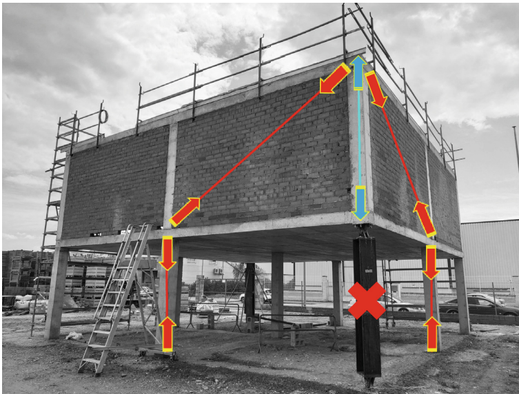
Fig. 7. Activation of an alternative load path based on the infill masonry walls.
