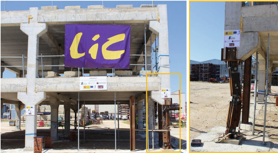
Fig. 10. Structure after the test.
