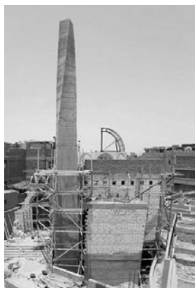
Figure 45_ Basuna Mosque Dome and its construction process (by Essam Arafa)
