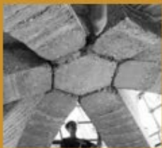
Rammed Earth dome: ETH students (BRG)
