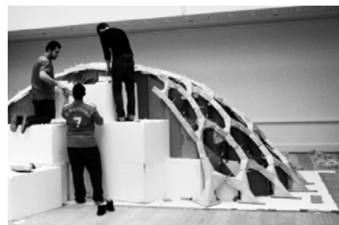
Figure 30_ Pre-Vault Pavilion and the extensive formwork needed (Larsen, Pedersen, and Pigram 2012) (Pedersen and Larsen 2015)
