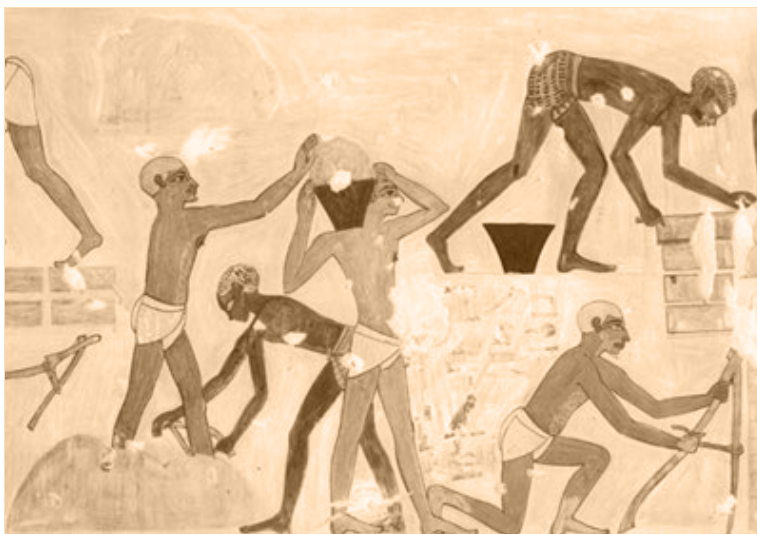
Figure 10_Mud brick at the time of the Ancient Egyptians. (Levantine Asiatics making bricks (Illustration from N. D. G. Davies, Paintings from the Tomb of Rekh-Mi-Rē [New York: Metropolitan Museum of Art, 1935], pl. 17)
