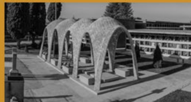
Tile Vault Construction
