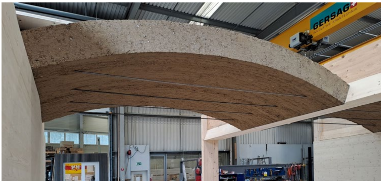
Figure 24_ Rammed earth segmental arch roof/ slab (Dietsche 2023)
