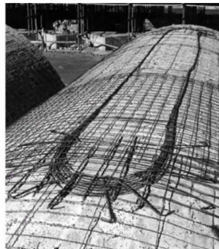
Figure 37_ Cristo Obrero Church roof layers prestressed (Warmburg 2017)
