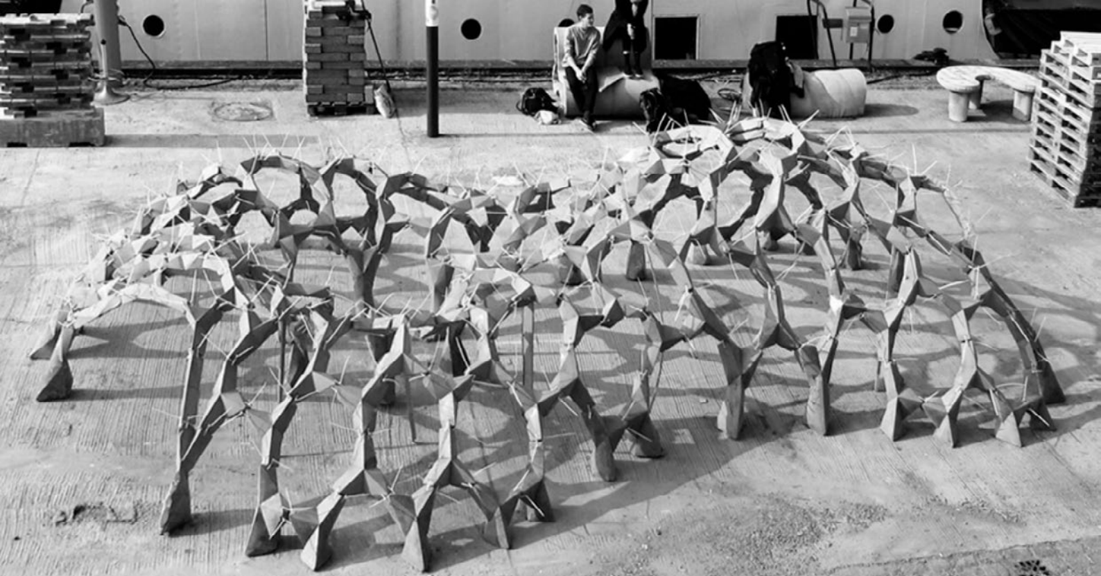
Figure 31_ A complex grid shell structure made up of 190 discrete concrete elements (Larsen and Pedersen 2013)
