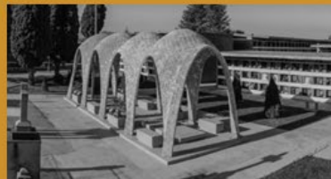
Tile Vault Construction
