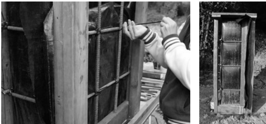
Figure 16_ Fabric mold for rammed earth (Lee 2021)
