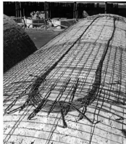
Figure 37_ Cristo Obrero Church roof layers prestressed (Warmburg 2017)
