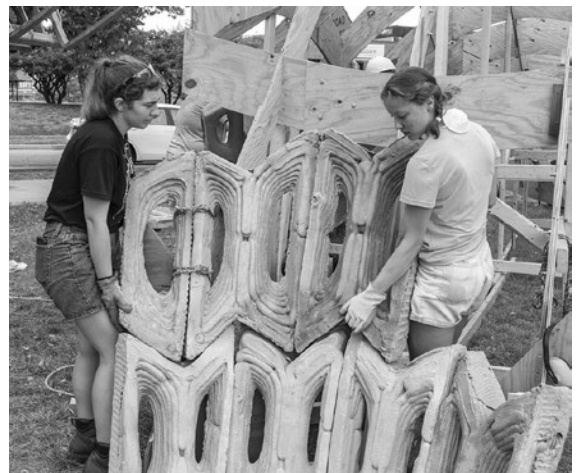
Figure 35_ Excessive formwork and different modules assembly. Photo by Hadley Fruits
