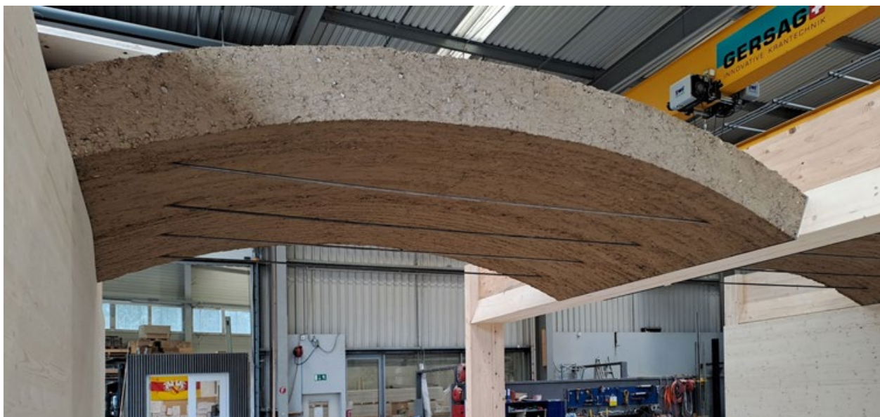
Figure 24_ Rammed earth segmental arch roof/ slab (Dietsche 2023)
