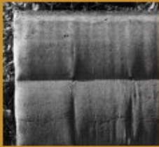
Fabric Formwork, Lee
