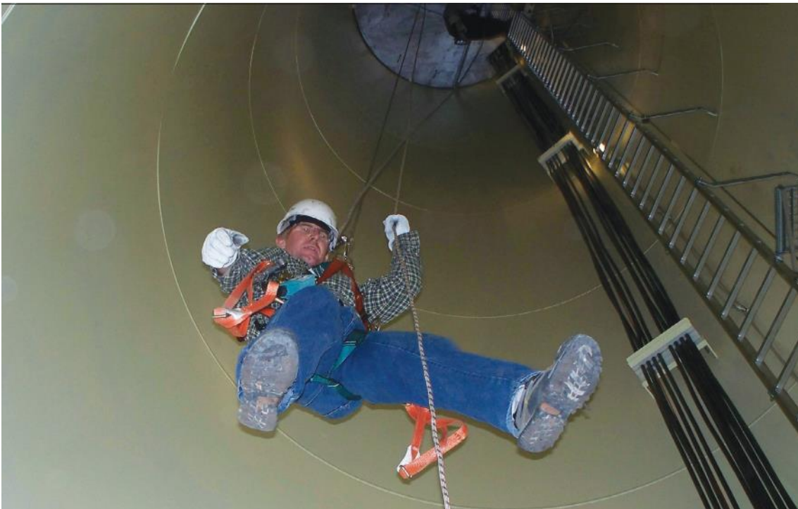
Fig. 10. A worker inside the turbine's tower (Source: (Atkinson, 2010))
