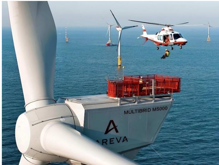
Fig 9. A helicopter transferring maintenance personnel to an offshore tower (Source: Tesicnor)
