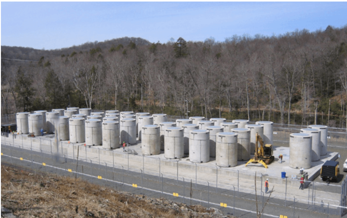
Figure 3.4: Dry cask intermediate storage at Connecticut Yankee [8].
